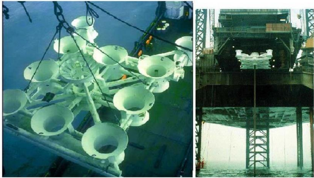
Figure 1.2 Nine slot template being lifted from a work boat (left) and being deployed from a drilling rig (right)[4].
