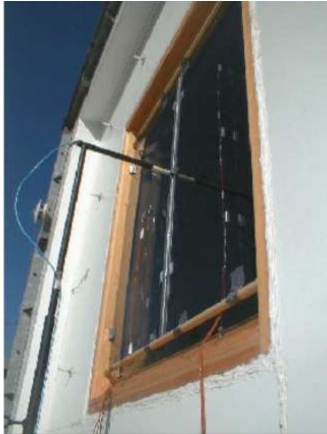
Figure 3.3 Image of the PASLINK test cell for the SOLVENT window
