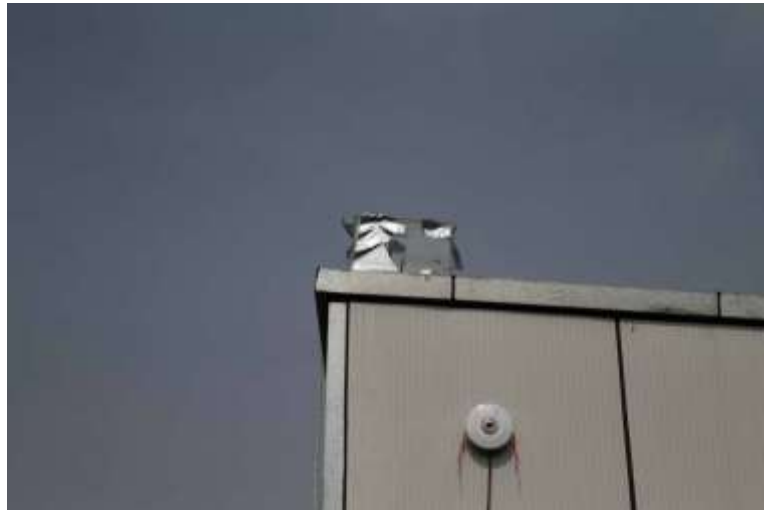
The outside luxmeter on the roof and the pyranometer on the east façade
