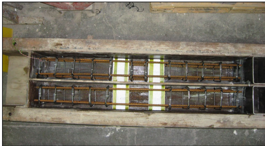
Figure 3-5: Steel moulds with reinforcement cages before casting
