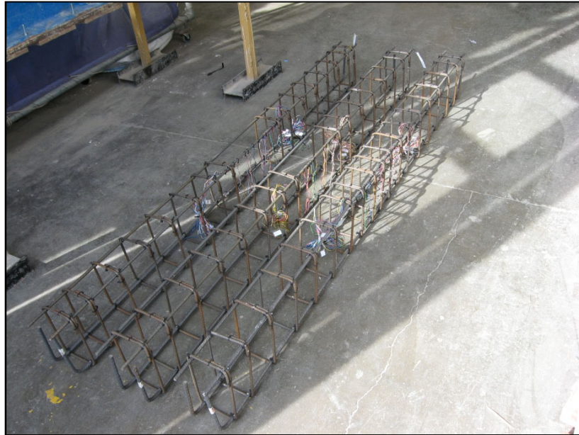
Figure 3-13: Completed reinforcement cages
