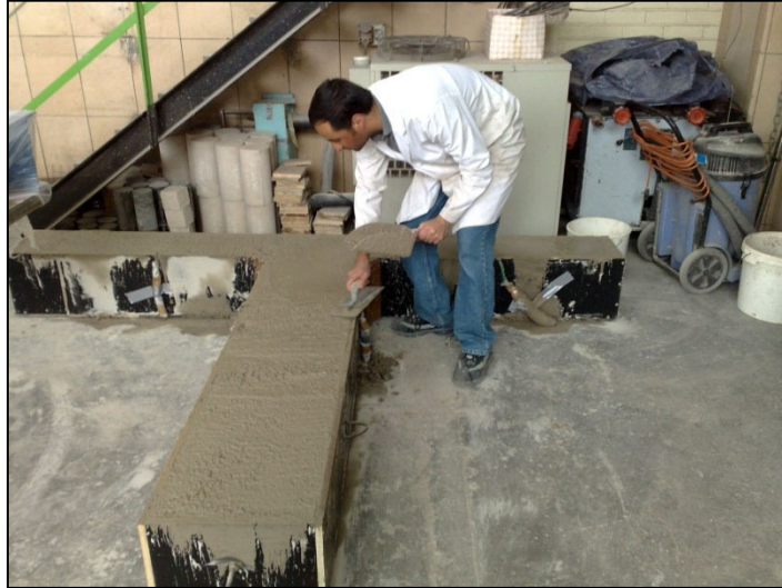
Figure 3-27: Casting and levelling of the specimen
