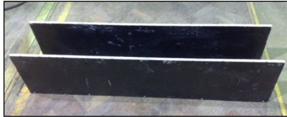
Figure 7-3: The formwork used for the repair
