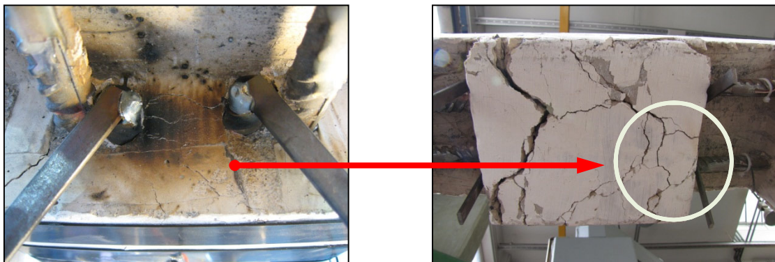
Figure 4-8: Formation of vertical splitting cracks and propagation along the splice (SC27-D16-PTMS1)
