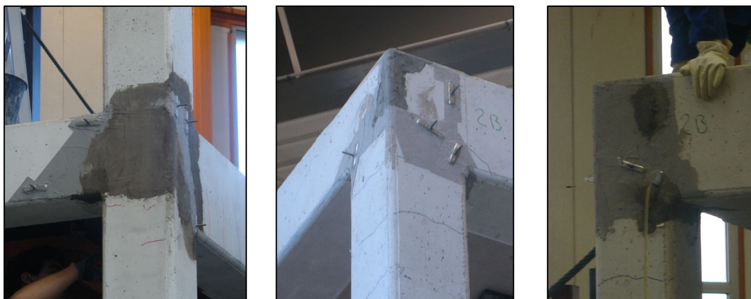
Figure 11-3(b): Joints after repair with new mortar
