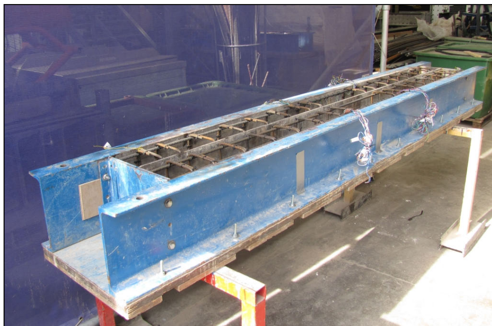
Figure 3-14: Beams ready for casting
