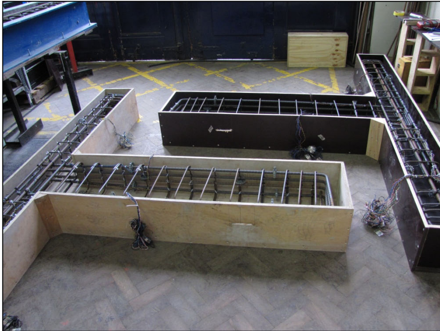
Figure 3-25: The cages positioned and tied in the formwork
