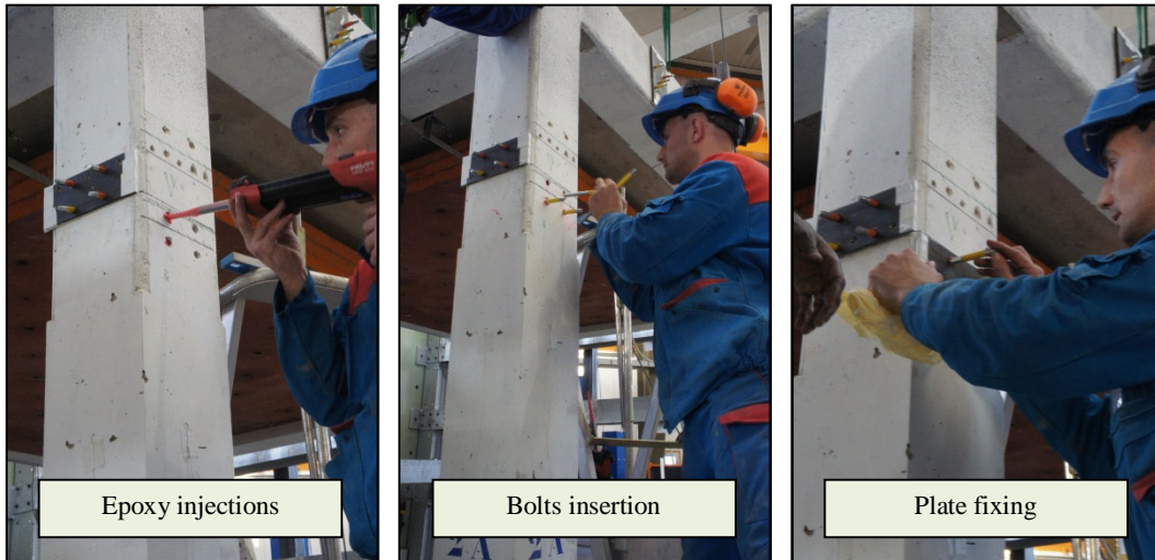
Figure 11-6: Stages of fixing the steel plates on a column side
