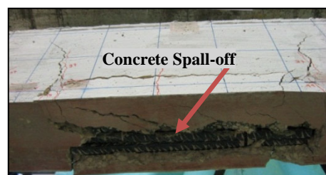
Figure 5-3: Spalling-off of the concrete cover in Specimen LC27-D16-Ctrl
