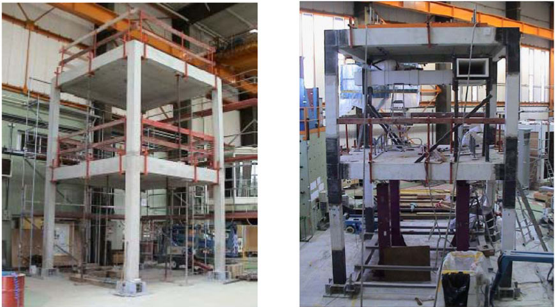
Figure 2-15: General view of the 2004 Saclay building (Chaudat et al., 2005)
