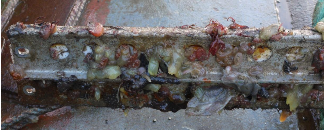
Figure 5.18. Back of panel holder in November 2012
