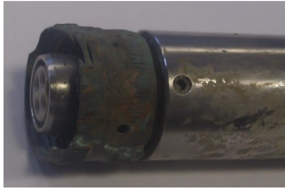
Figure 9.3. Corrosion of outer ring of FO connector
