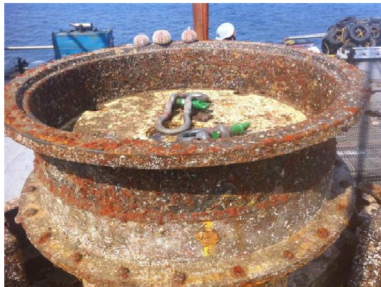
Figure 4.35. Flange at top of dummy foundation prior to cleaning
