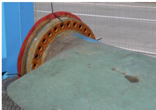
Figure 4.25. Corrosion observed around blade fixings
