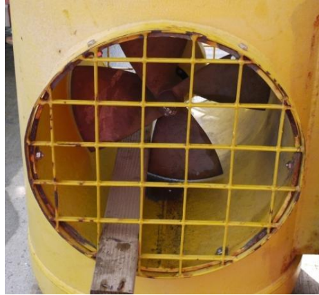
Figure 4.34. Corrosion due to coating removal around rim of thruster opening
