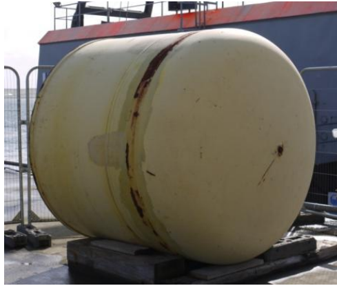
Figure 4.22. Buoyant nose showing signs of corrosion around the circumference
