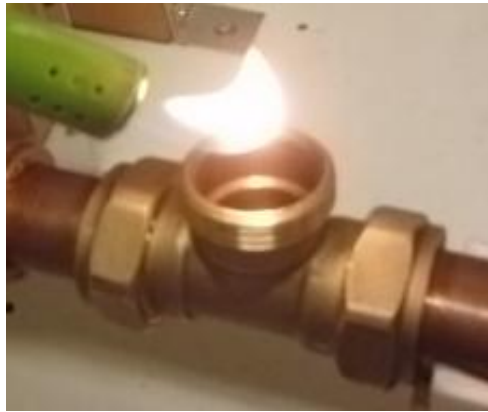
Figure 3.4 Gas lighter ignition
