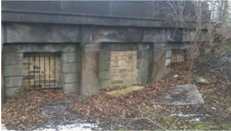
Figure 65: Old Entrance to the Undercroft
