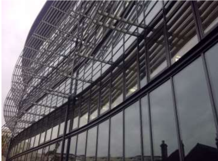
Figure 36: South Side of the Ziff Building
