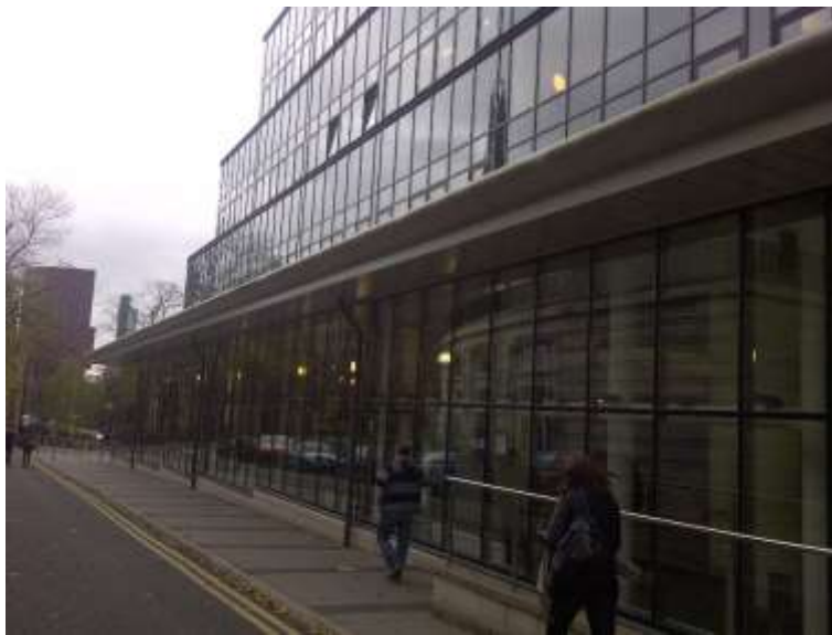
Figure 35: North Side of the Ziff Building
