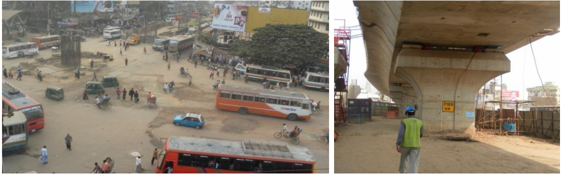
Figure 5.11: Flyover and its pillars at Sayedabad location
