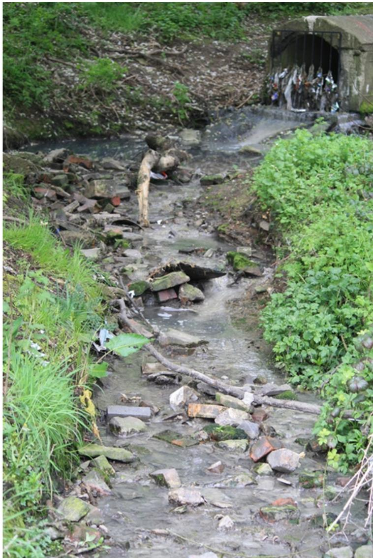
Figure 6.1: A surface water outfall showing significant aesthetic indicators of misconnection pollution, Tongue gutter, Parson Cross, Sheffield.
