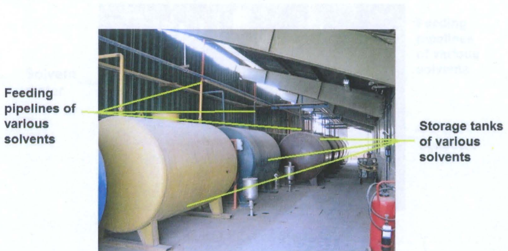
Figure 2.19 Solvent storage tanks of the resin plant
