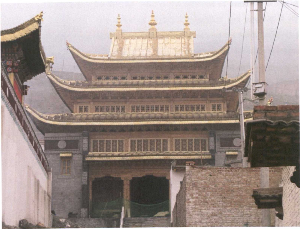
Figure 5.10 Rongwo 1,000 Buddha images temple under construction, summer 2009
