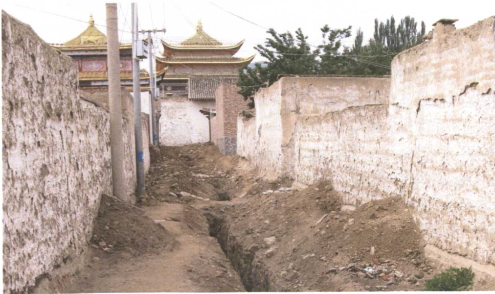
Figure 5.9 Work at Rongwo to lay new water pipes
