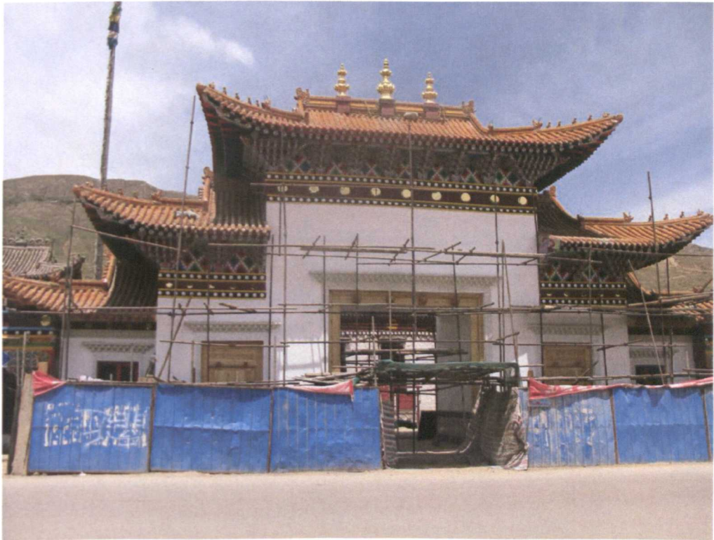
Figure 5.3 Rongwo ticket gate under construction, early summer 2009
