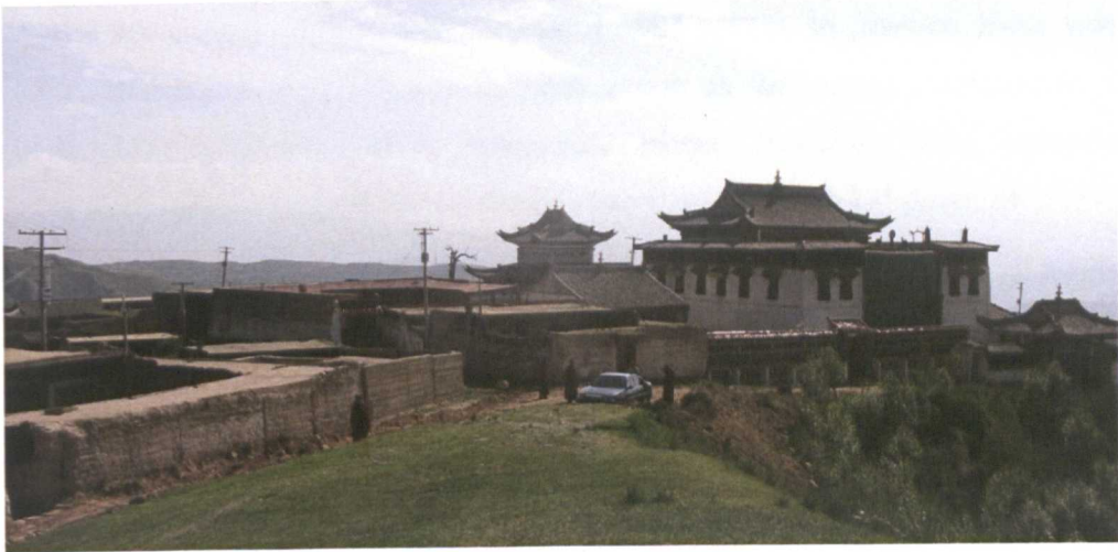
Figure 3.2 Tashikhyil's rebuilt assembly hall
