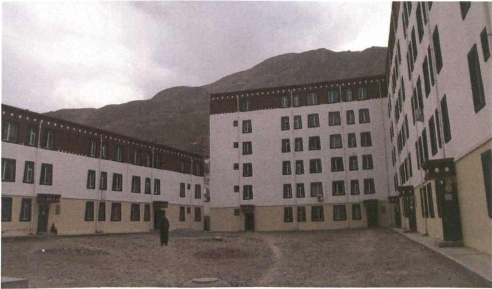
Figure 5.8 New housing on Chorten Khamtsen site
