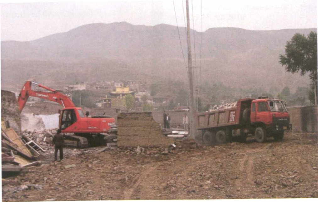
Figure 5.7 Demolition of Chorten Khamtsen, Rongwo
