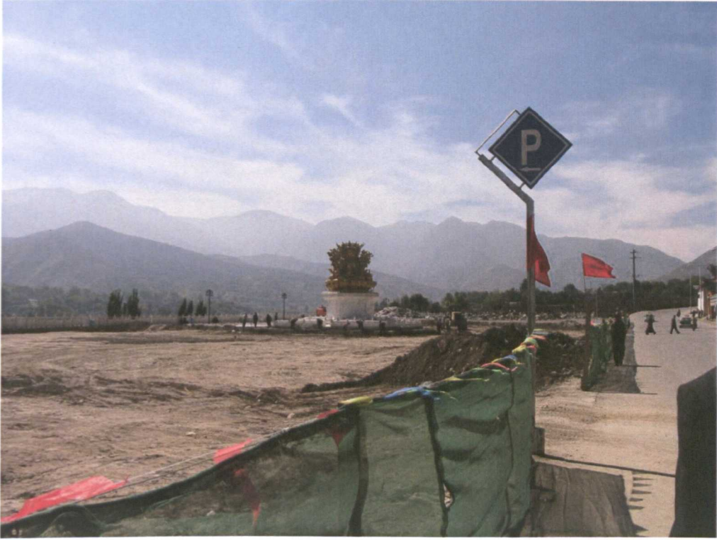
Figure 5.2 Rongwo cultural square under construction, autumn 2008
