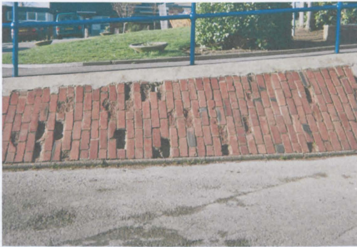
Figure 7.10 – Playground Wall, Holy Cross
