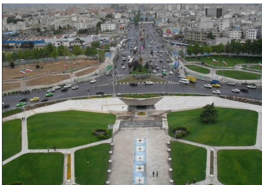
Figure 21: The pedestrian entrance on the eastern edge. The picture also shows the water pools that were inspired by Iranian Gardens, Source: ("Symbol of Tehran," 2011)
