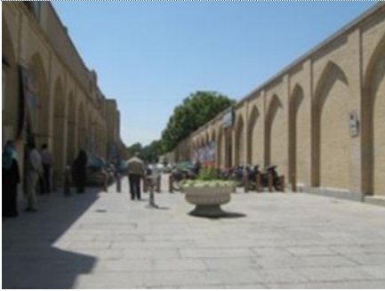
"Bollards prevent car access"
