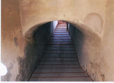
⚡ this sector has distinct character with this roofed pathway
