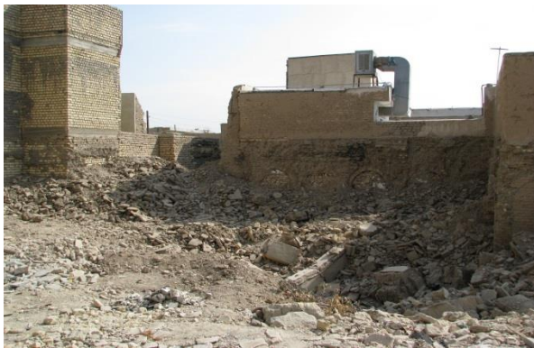
Picture 22: ruined area
