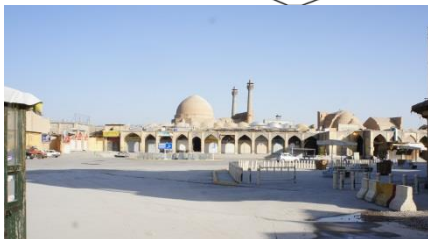
Photo 1: from part 38 shows the Jameh mosque of Isfahan which is an important historic building which gives a striking image to this space
