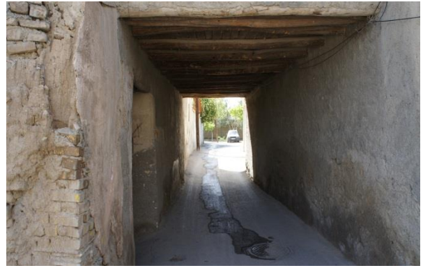
Picture 21: roofed pathways
