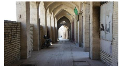
Photo 2: from part 3 and shows the really narrow part just for pedestrian movement
