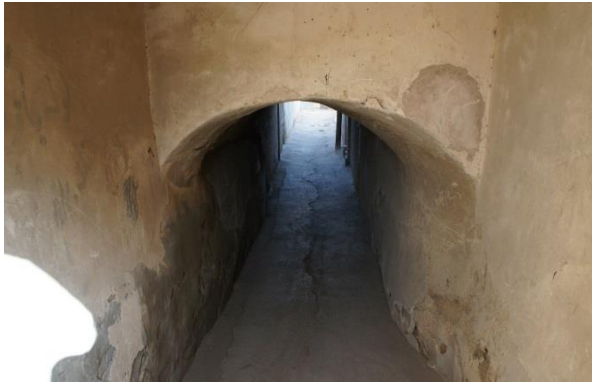
Picture 20: roofed pathway
