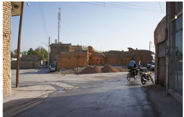
Picture 23: ruined area
