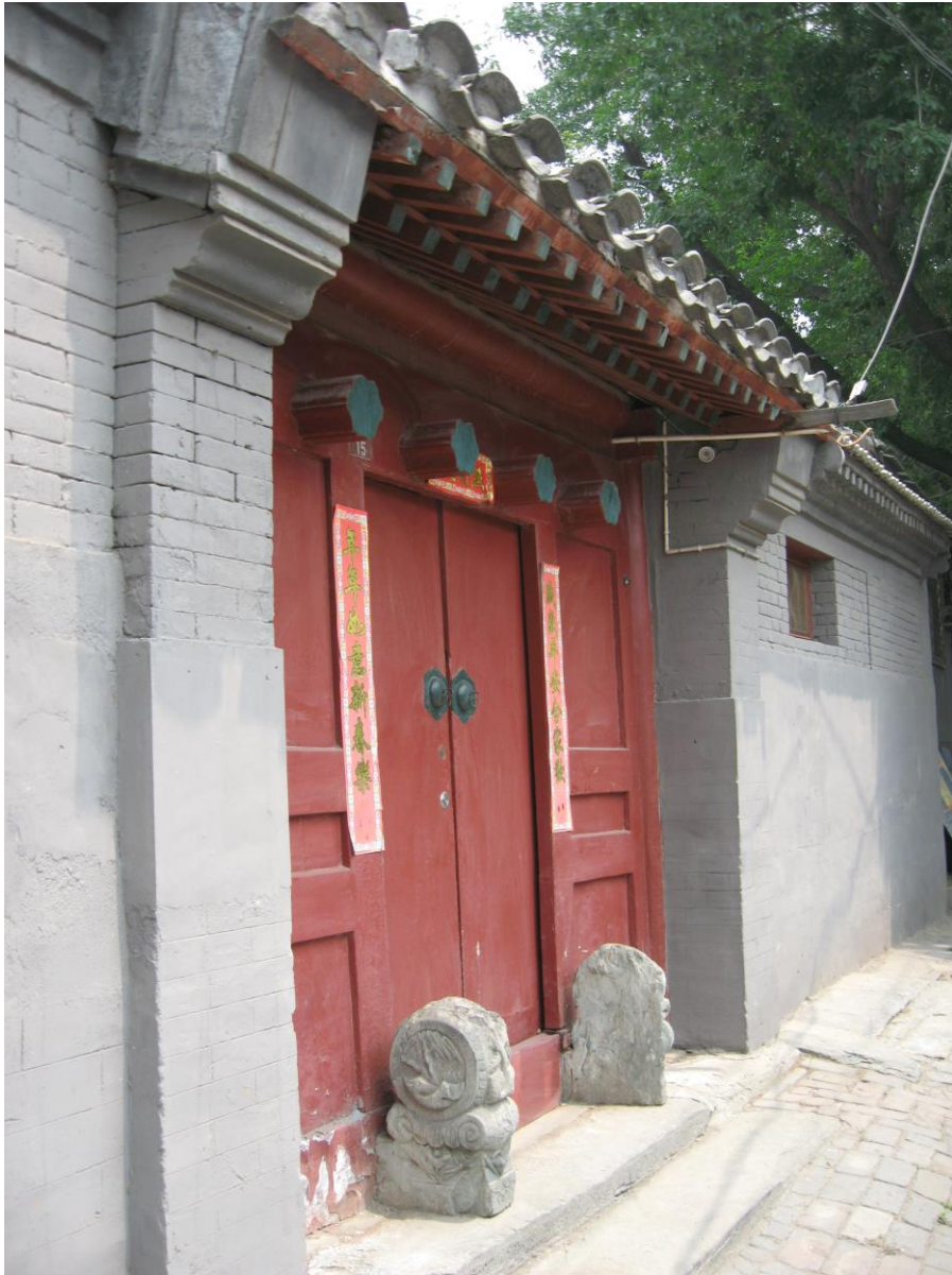
Figure 3-23 The Main Gate of 15 Hou Dram Tower Yuan Alley. Source: Photo taken by Bing Jiang, 2007. A humble gate of a common si-he-yuan residence, with a simple roof over the doorway.
