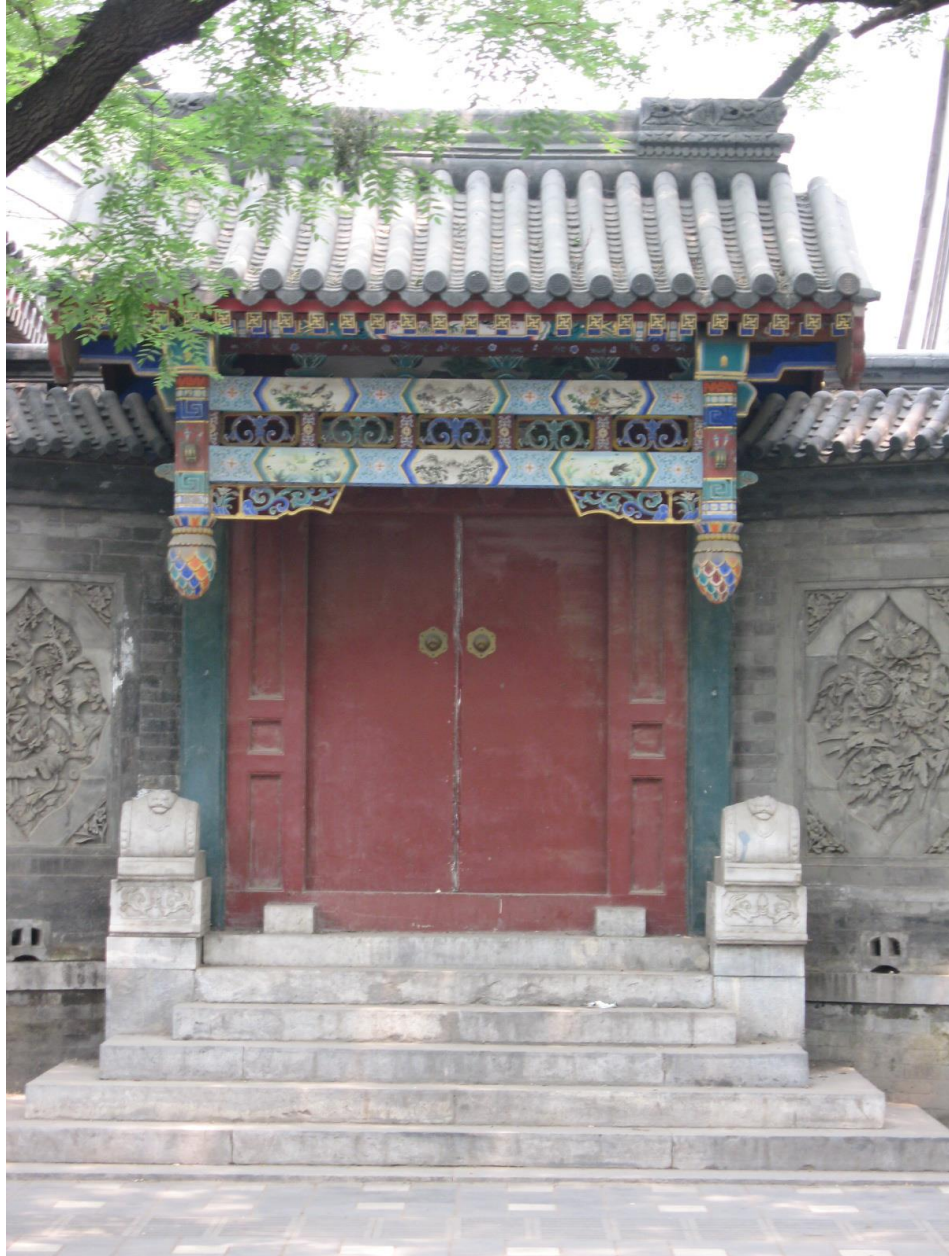
Figure 3- 24 The Second Gate of a Si-he Courtyard Compound: chui-hua-men . Source: 05 Beichizi Street, Beijing, photo taken by Bing Jiang, 2007. The gate is built up higher than the courtyard ground, with several steps and a roof over it. The decorations under the roof are elaborate.
