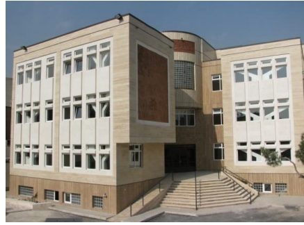
Figure 2.12: South façade of Zeinab School
