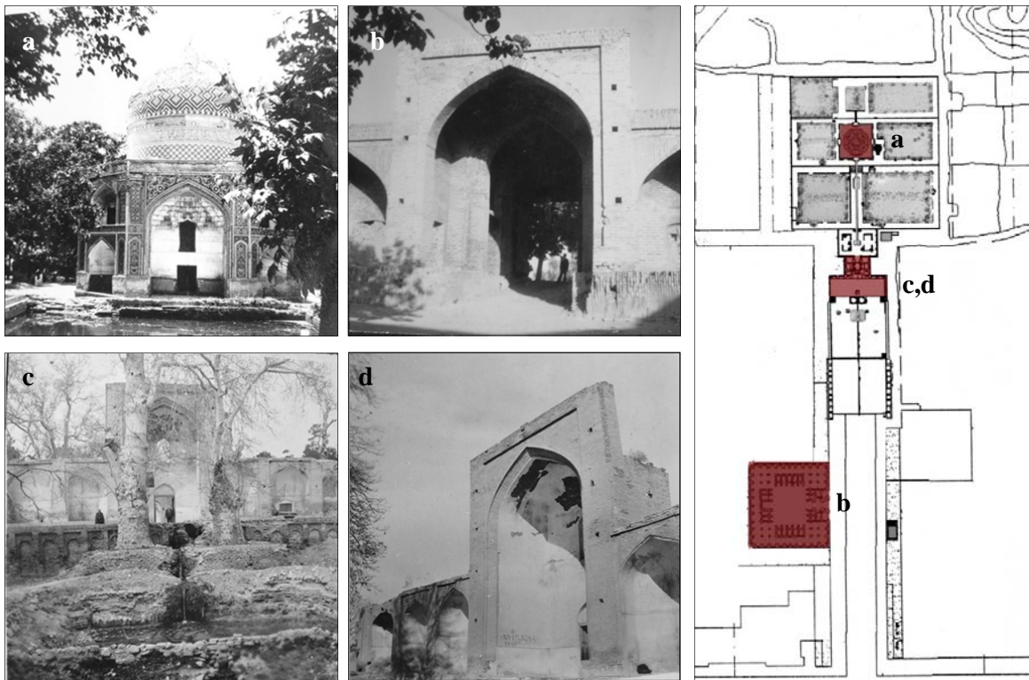
Figure 5.7: Material deterioration of Qadamgah during the Pahlavi era and their location on the map, (Source of photos Courtesy of the Document Centre of the ICHHTO, branch of Khorasan-e- Razavi, Mashhad, Source of map: Highlights and numbers added by the author)
