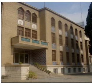
Figure 3.28: Above Left: General view of Narenjestan before its demolition, (Source: Album of Photographs by Ali Khan Vali, p.287); Above right and below: general view and plan of Khabgah-e-Elizeh, constructed in 1342 SH/1963, (Source: Courtesy of the Technical office of the Golestan palace)
