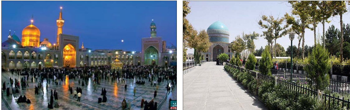
5.1: Right: Holy Shrine of Imam Reza in Mashhad ;Left: Tomb of Khaje Rabi in Mashhad, (Source: Fras News Agency, photo by Armin Kermani)
