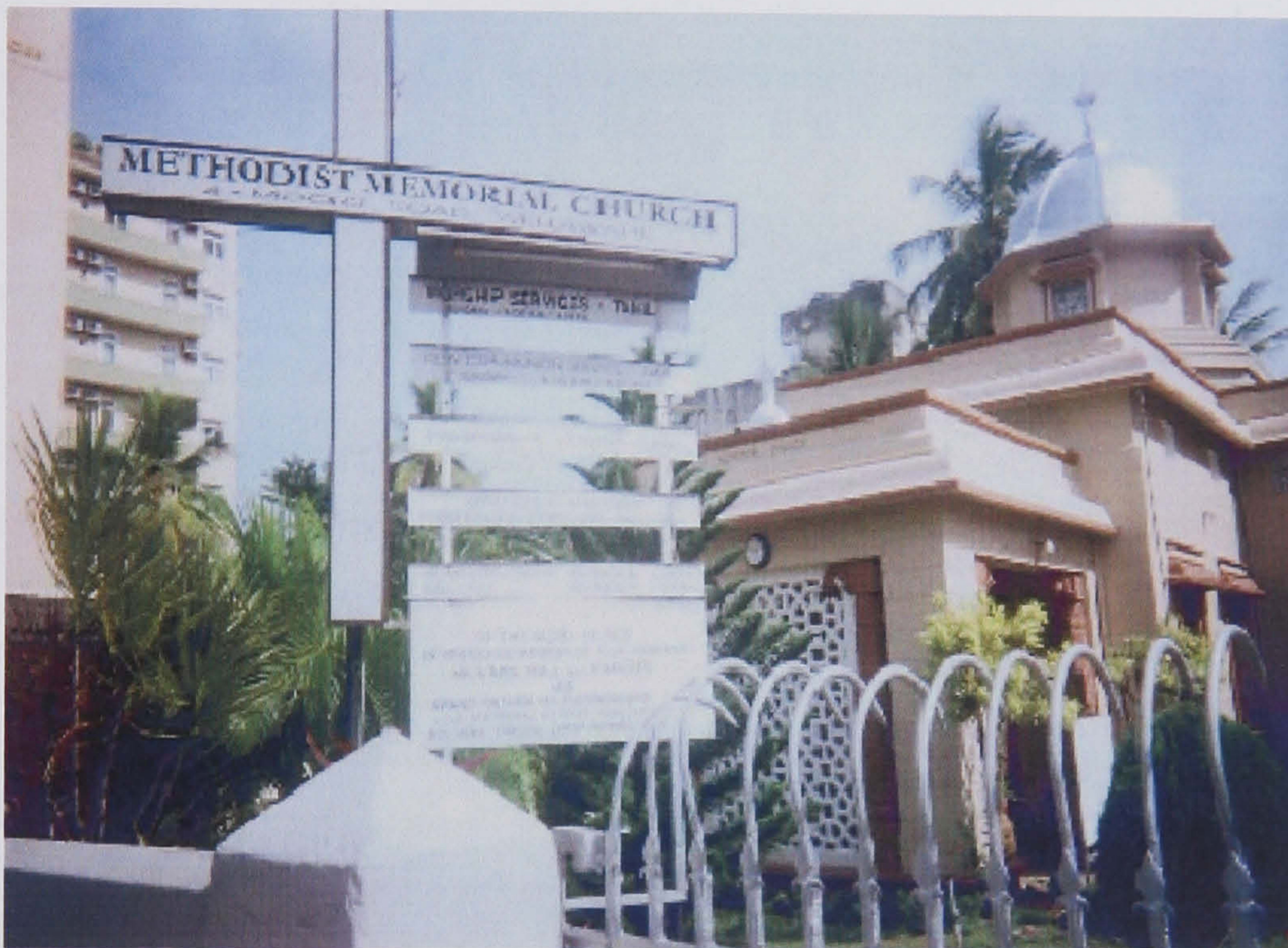
Plate 3. Moor Road Methodist Church – The site of a number of interviews in Colombo 7
