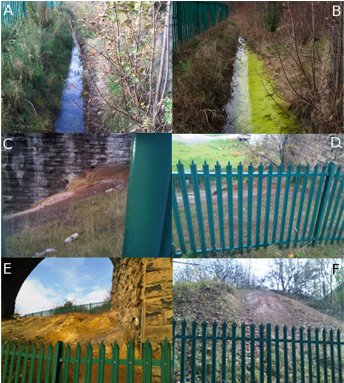
Figure 2.7: (A) and (B) show the drainage ditch to the south of the site at differing times of the year. (C), (D), (E) and (F) show the exposed COPR waste which has been fenced off to stop public ingress.
