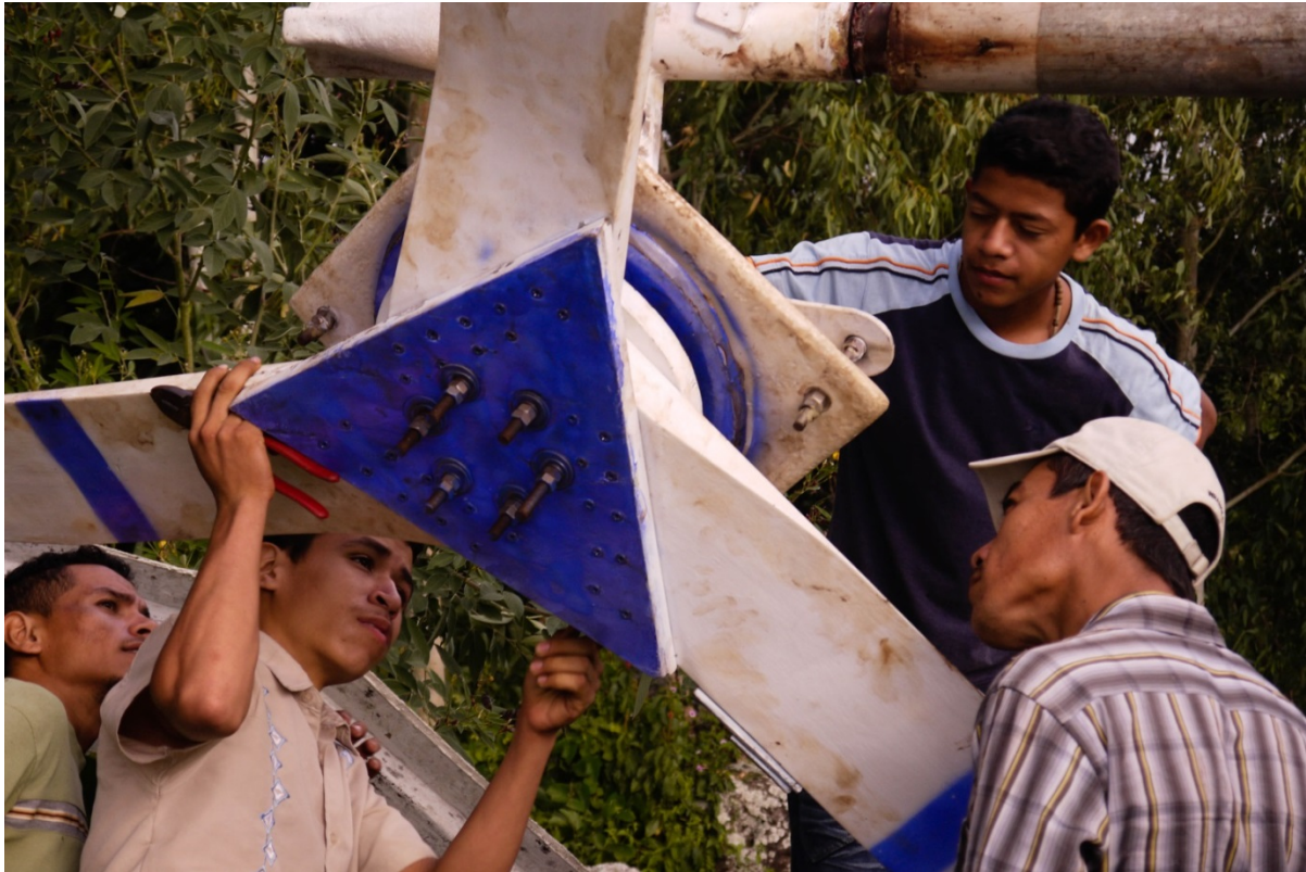
Figure 5-18: Inspection of the rotor and stator by the Cuajinicuil technicians to prevent a potential future failure.
