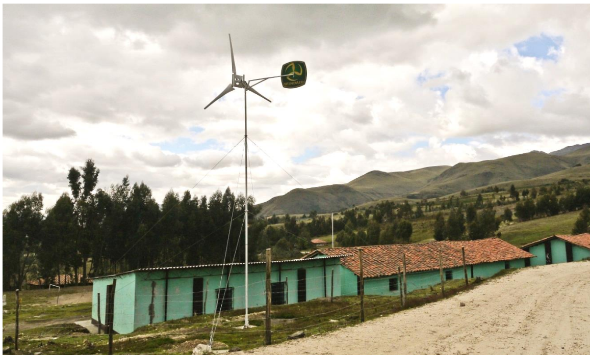
Figure 4-10: WindAid's 2.5kW turbine installed at La Florida in the Huamachuco area.
