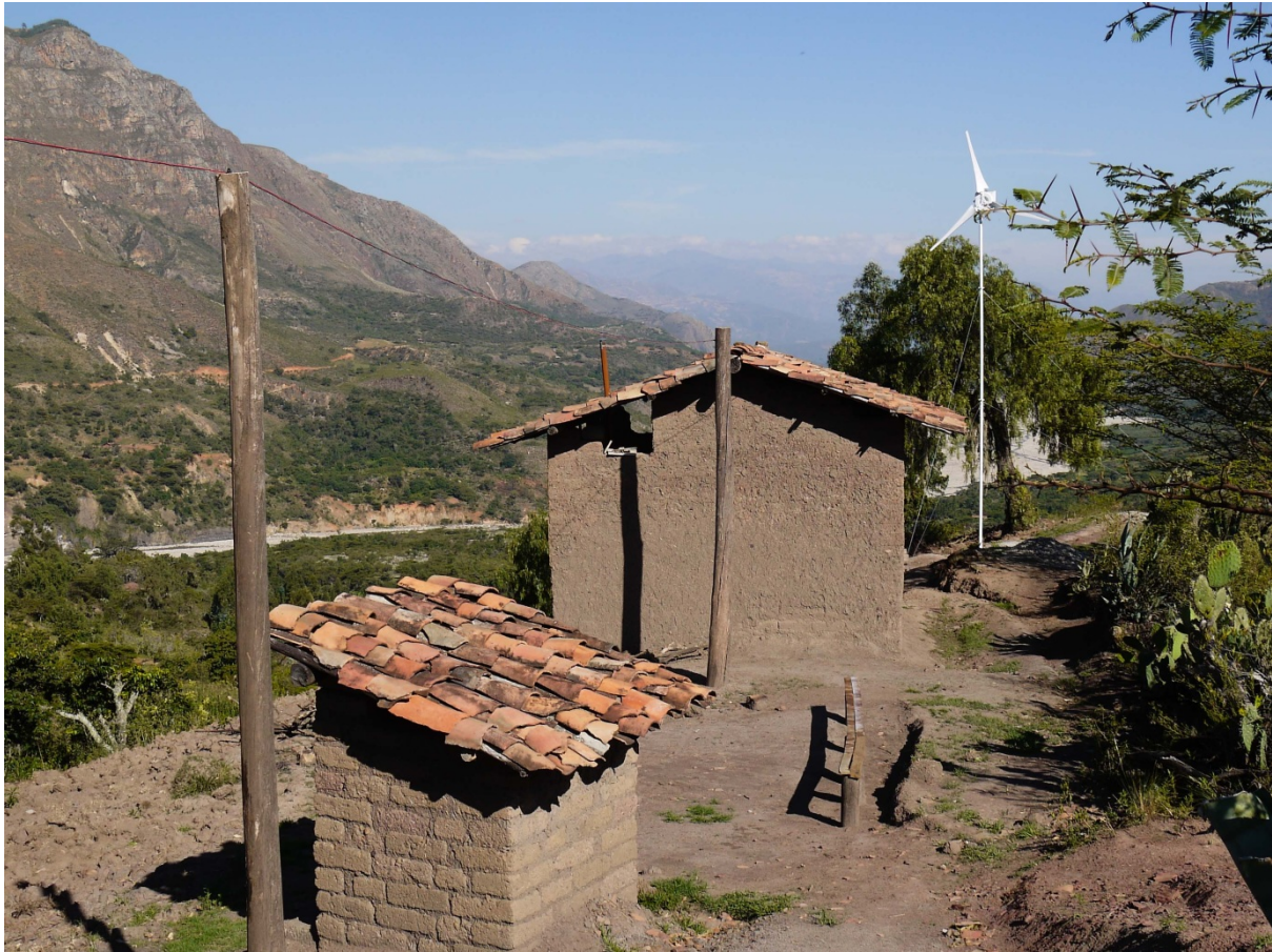
Figure 4-16: Wind turbine installed by WindAid at El Olivo on a ridge, but between a tree and the powerhouse.
