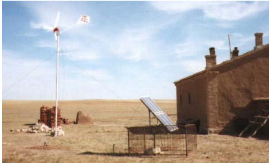
Figure 2-12: Wind/PV demonstration system (Batchelor et al. , 1999).
