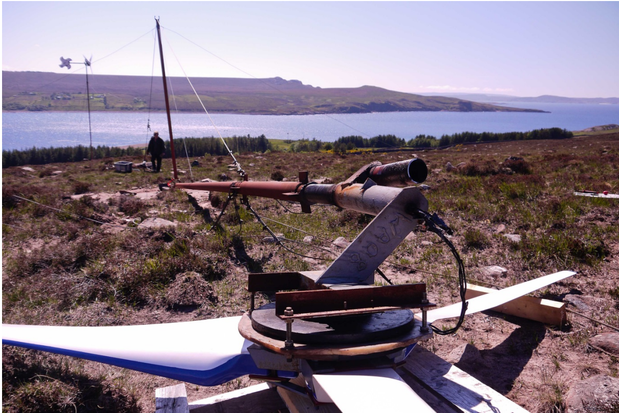
Figure A-8: a) Lowering Athini's SWT for maintenance and b) resting the turbine on the ground for inspection.
