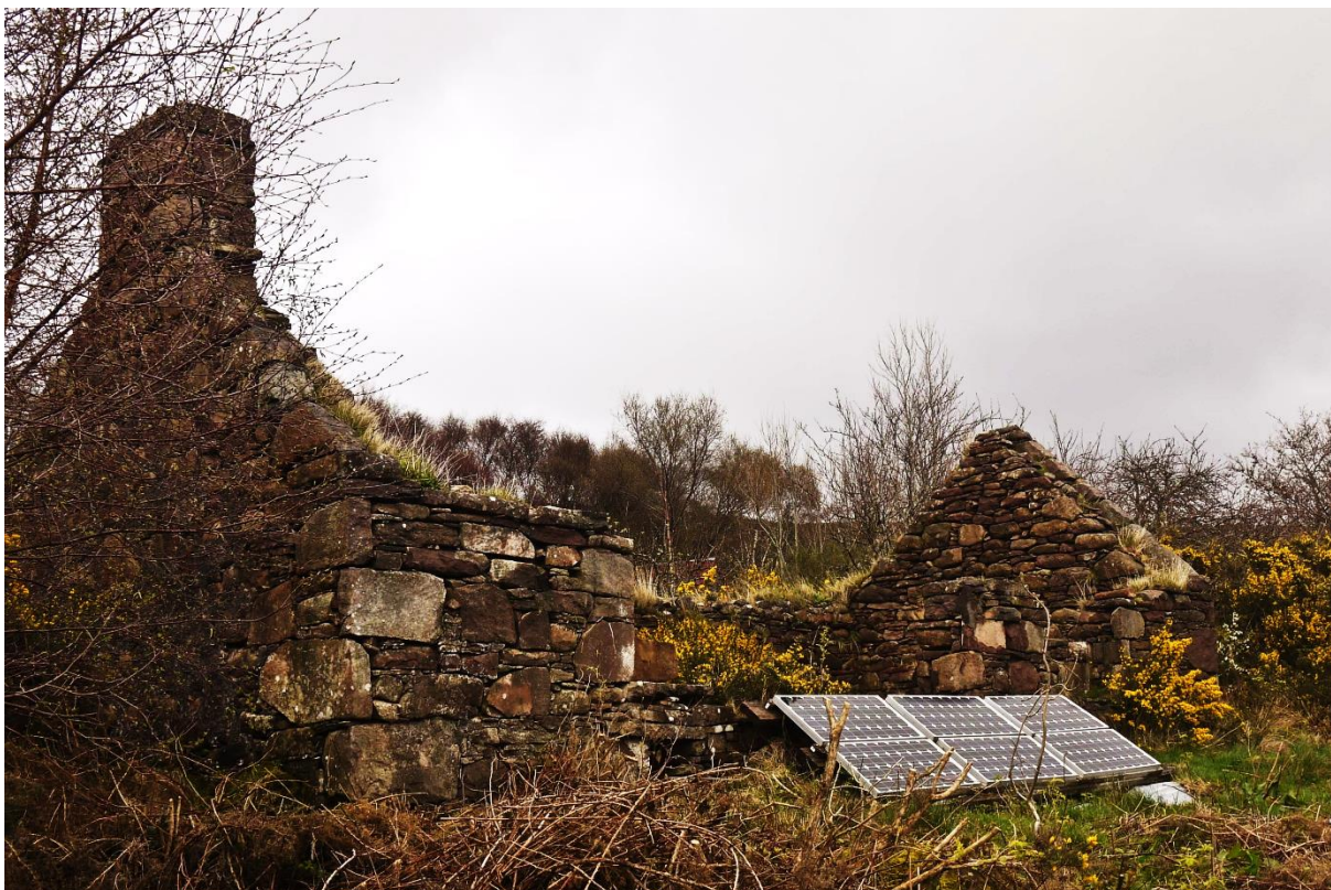
Figure 6-17: A renewable energy upgrade to one of the original stone crofting cottages.
