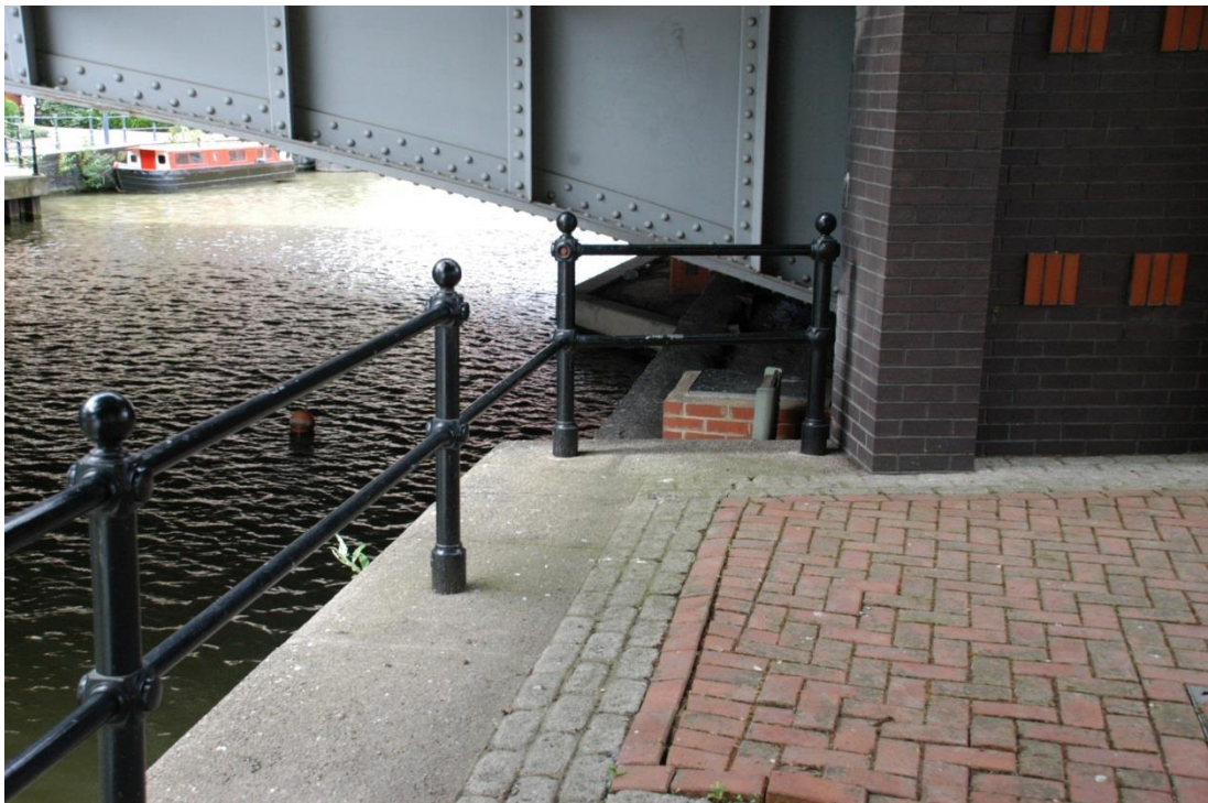
Figure 48 - entrance to 'Under the Bridge' with rung missing, Bristol (photo: author's own)
