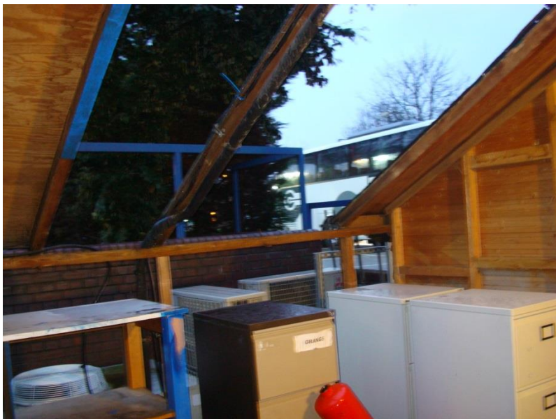
Figure 31 - roof removed from Ramada hotel bin store, Bristol (photo: author's own)
