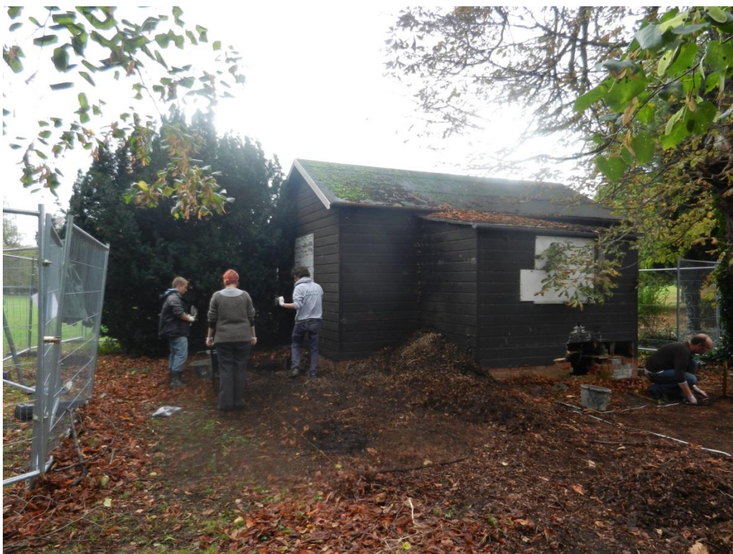
Figure 67 - 'The Cricket Pavilion', Bootham Park Hospital grounds, York (photo: author's own)
