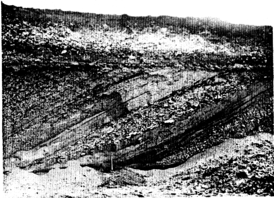
Plate 25. Prescott's Pit (Elloughton Quarry South) on the 20 m terrace showing cross-bedded gravels dipping towards the south east at about 45° overlain by horizontally bedded gravels. Note the truncated top to the cross-bedding. The section, which is about 4.5 m high, is located at SE 932 288 (Fig. 17). Photograph from Sheppard (1897).
