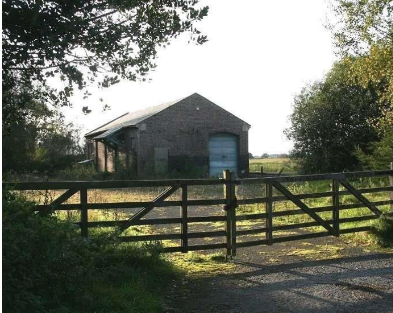
Figure 4. Ganton goods shed, showing the awning on the roadside. Courtesy of John Furnevel.
