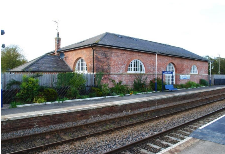
Figure 22. Hutton Cranswick goods shed viewed from the Up platform.
