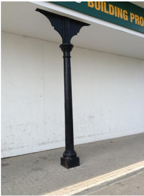
Figure 17. One of the cast iron columns at Pocklington.
