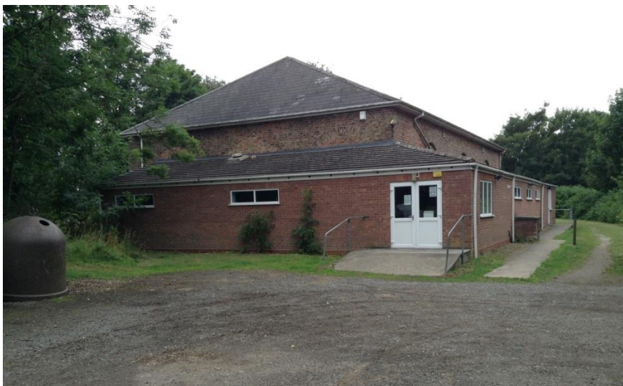
Figure 10. The roadside and extension on Stamford Bridge goods shed.
