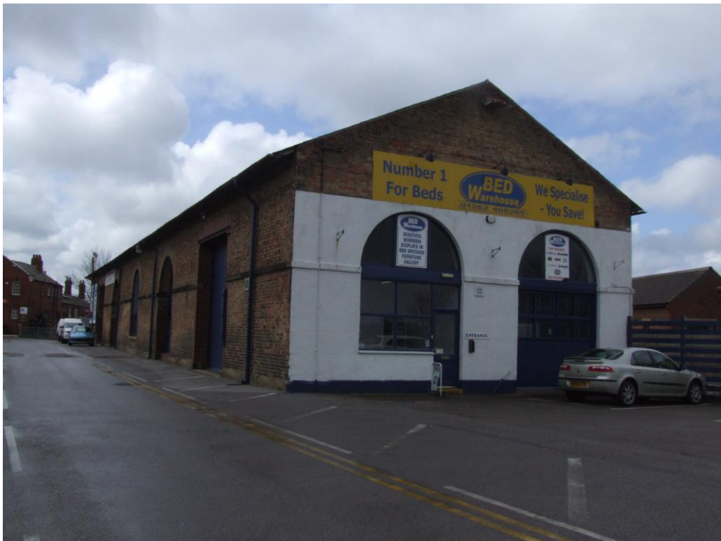
Figure 36. Bridlington goods shed as it stands today. Picture courtesy of Chris Tommis.
