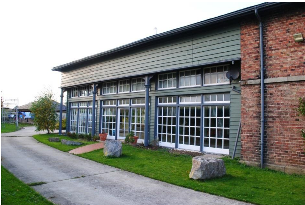
Figure 32. The loading bay at Nafferton, with weatherboarding and new entrance in the glazed side.
