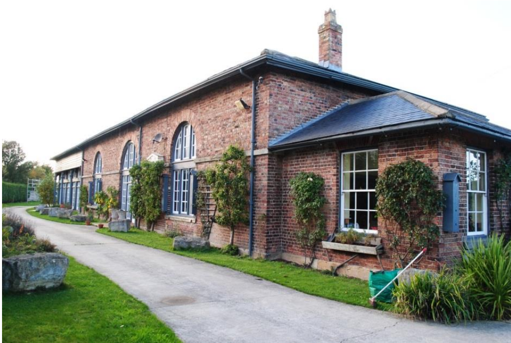
Figure 31. Nafferton goods shed road side view with the office and loading bay visible.
