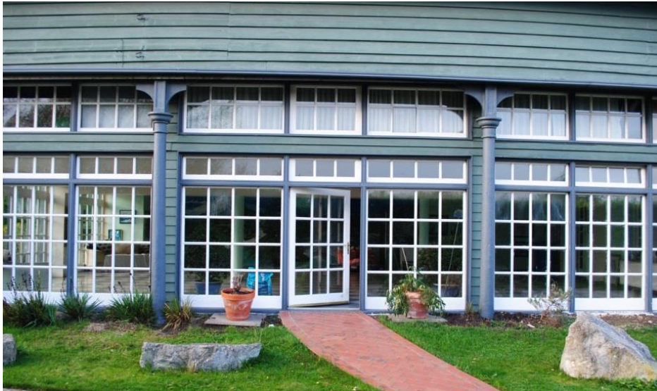
Figure 33. The new side entrance in the loading bay.
