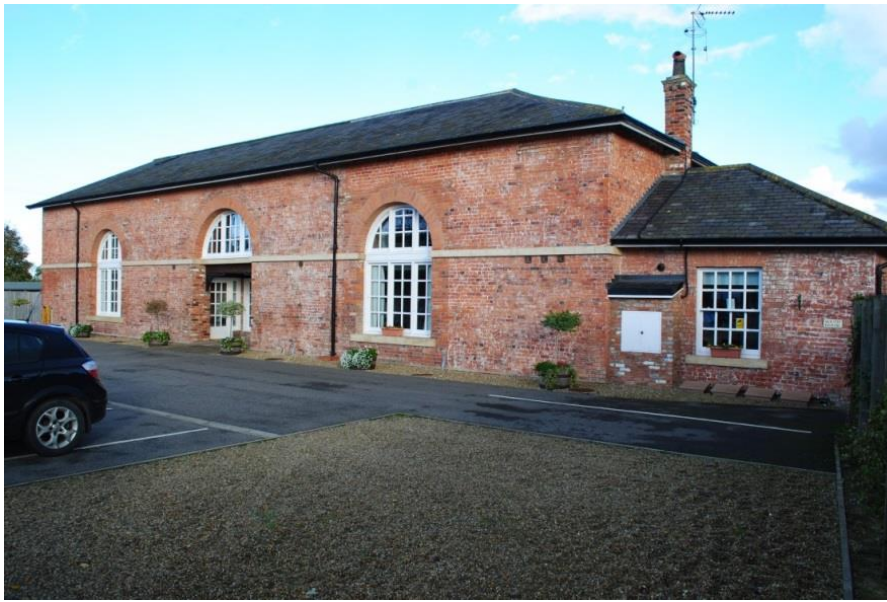
Figure 23. The road side of hutton Cranswick goods shed, with new meter box visible.
