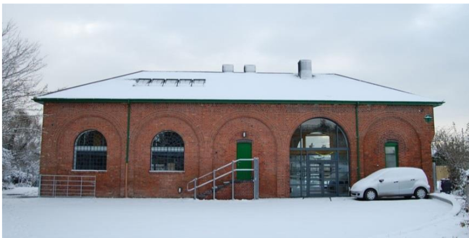
Figure 40. The goods shed at Wareham, showing arches and hipped roof. Courtesy of Morgan Carey Architects.
