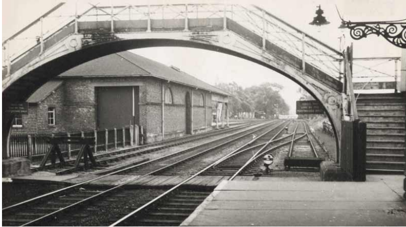
Figure 14. A view of Pocklington goods shed in 1965 showing the weather-boarded loading bay and railway side rounded door. Copyright of William Fawcett and courtesy of www.railwayarchitecture.org.uk .
