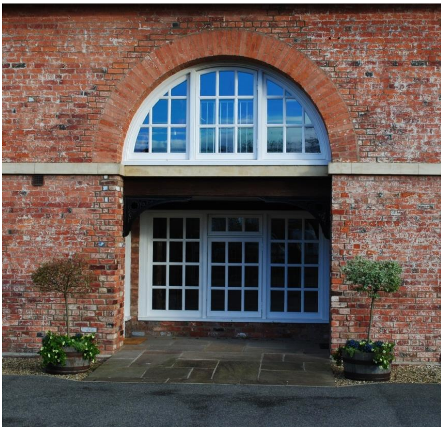
Figure 24. The road side door, with new metal brackets beneath the original stone course.
