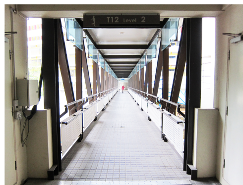
View of deck from Block T12A
