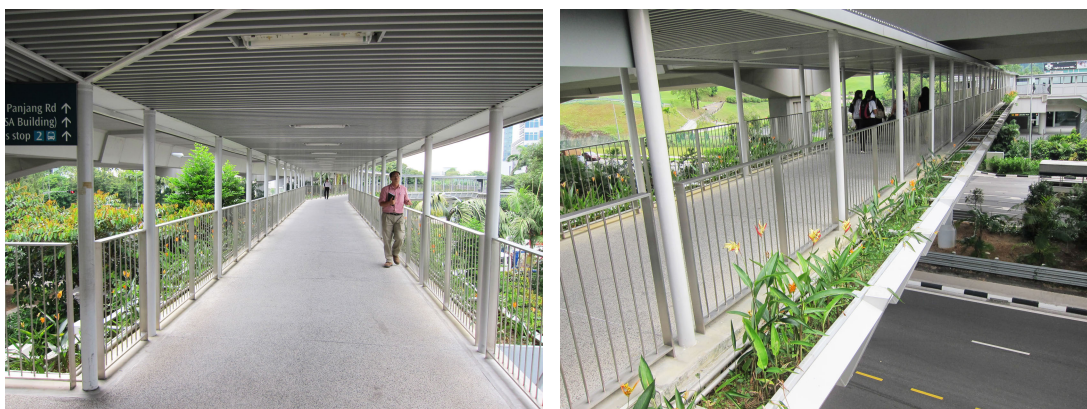
Figure 6-28. The POB deck, roof and planters of spans T4 (left) and T5 (right).
