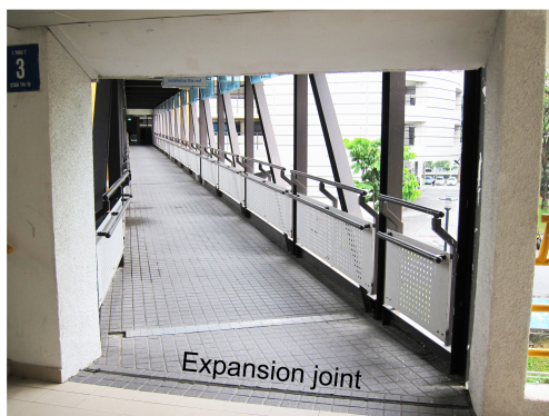
View of deck from Block T15
