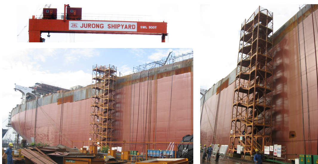
Figure 4-6. The gantry tower used as a test structure at the Jurong Shipyard in Singapore.
