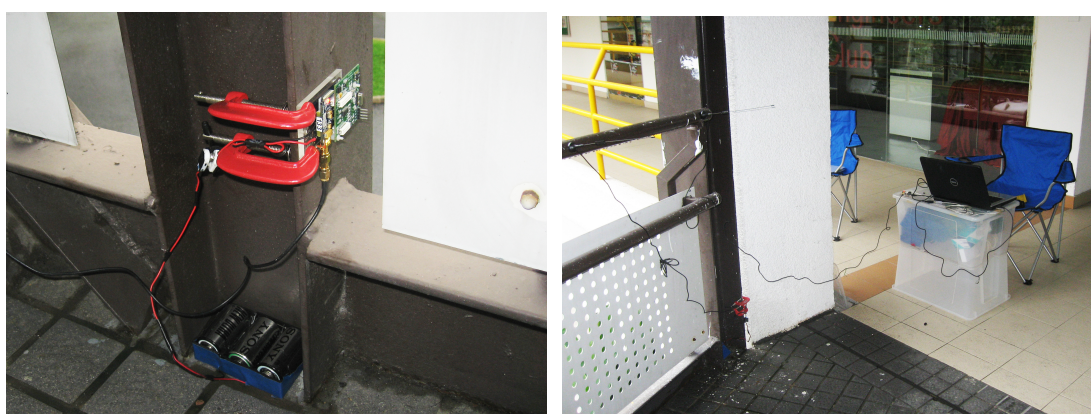
Figure 4-18. One of the sensor nodes clamped to the column (left) and the sensor node and base station at the cantilever end of the footbridge (right).
