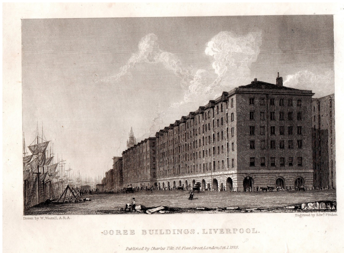
Figure 28: Goree Buildings, Liverpool, (1826) engraving by Edward Finden, scan of engraving copy owned by author.
