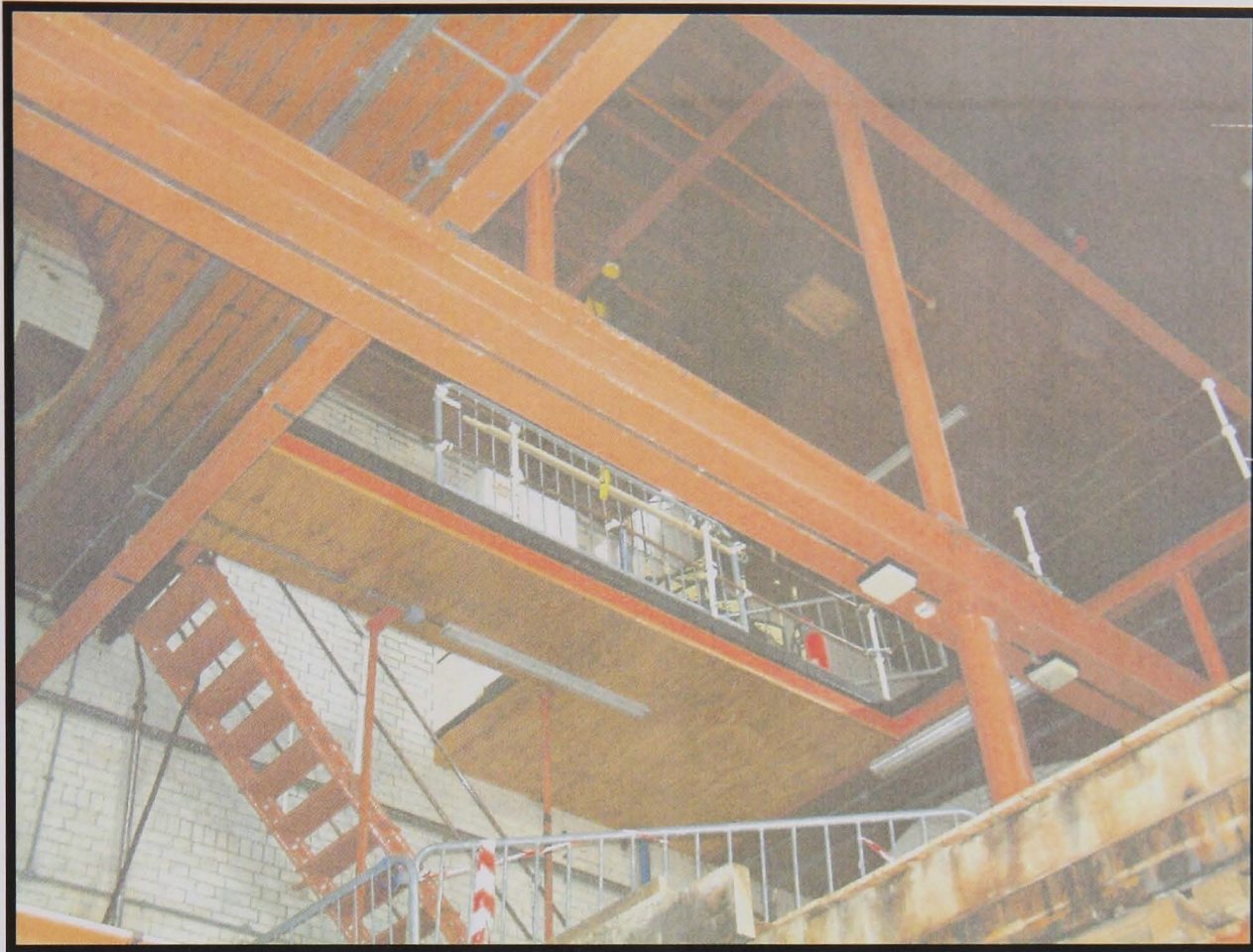
Figure 11: Inside the Main Brewhouse, Source: Hotel Architect
