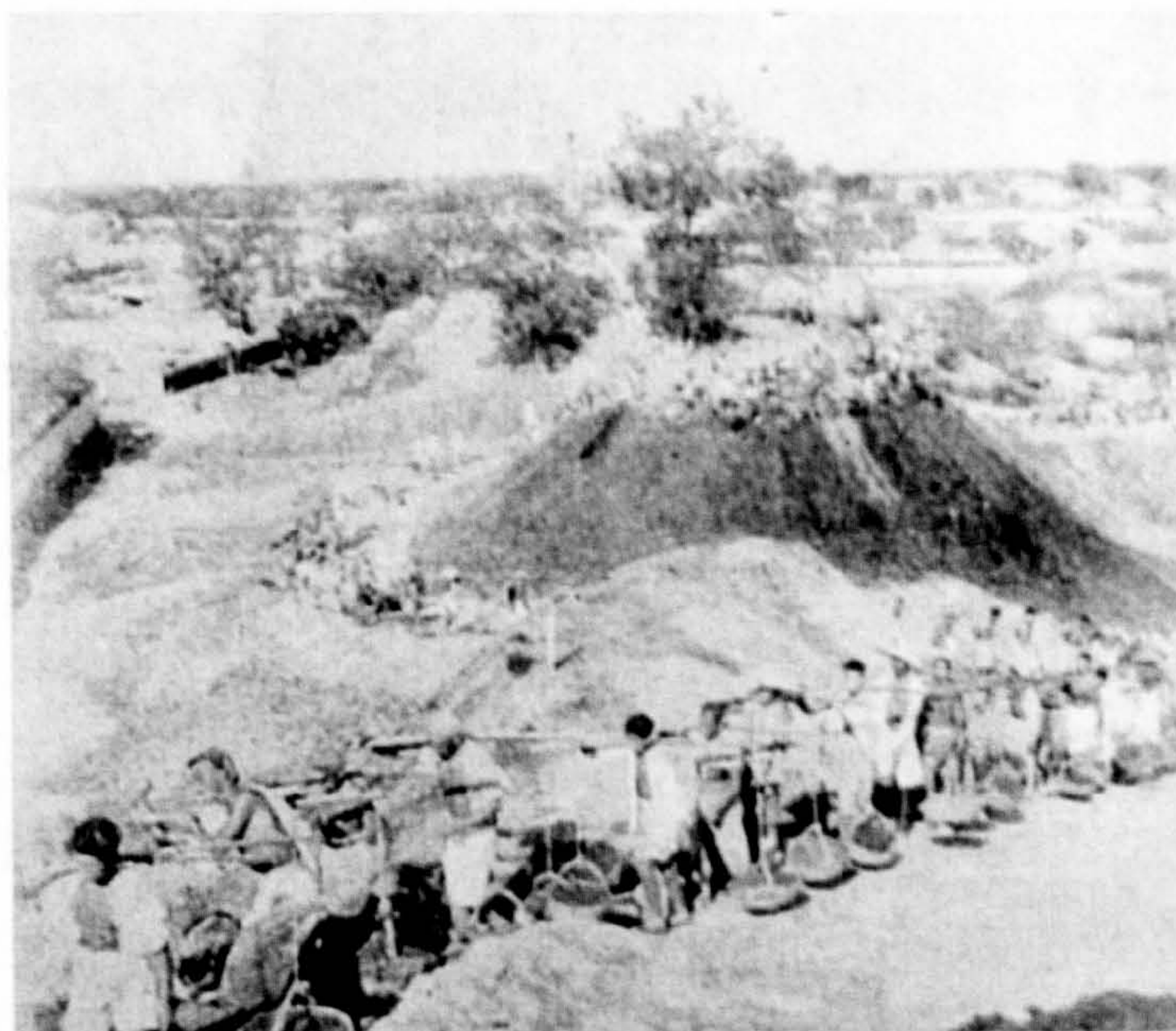
Figure 3.3 Digging and mounding project with mass manual volunteers for the creation of Joyous Pavilion Park, Beijing, in 1952.
