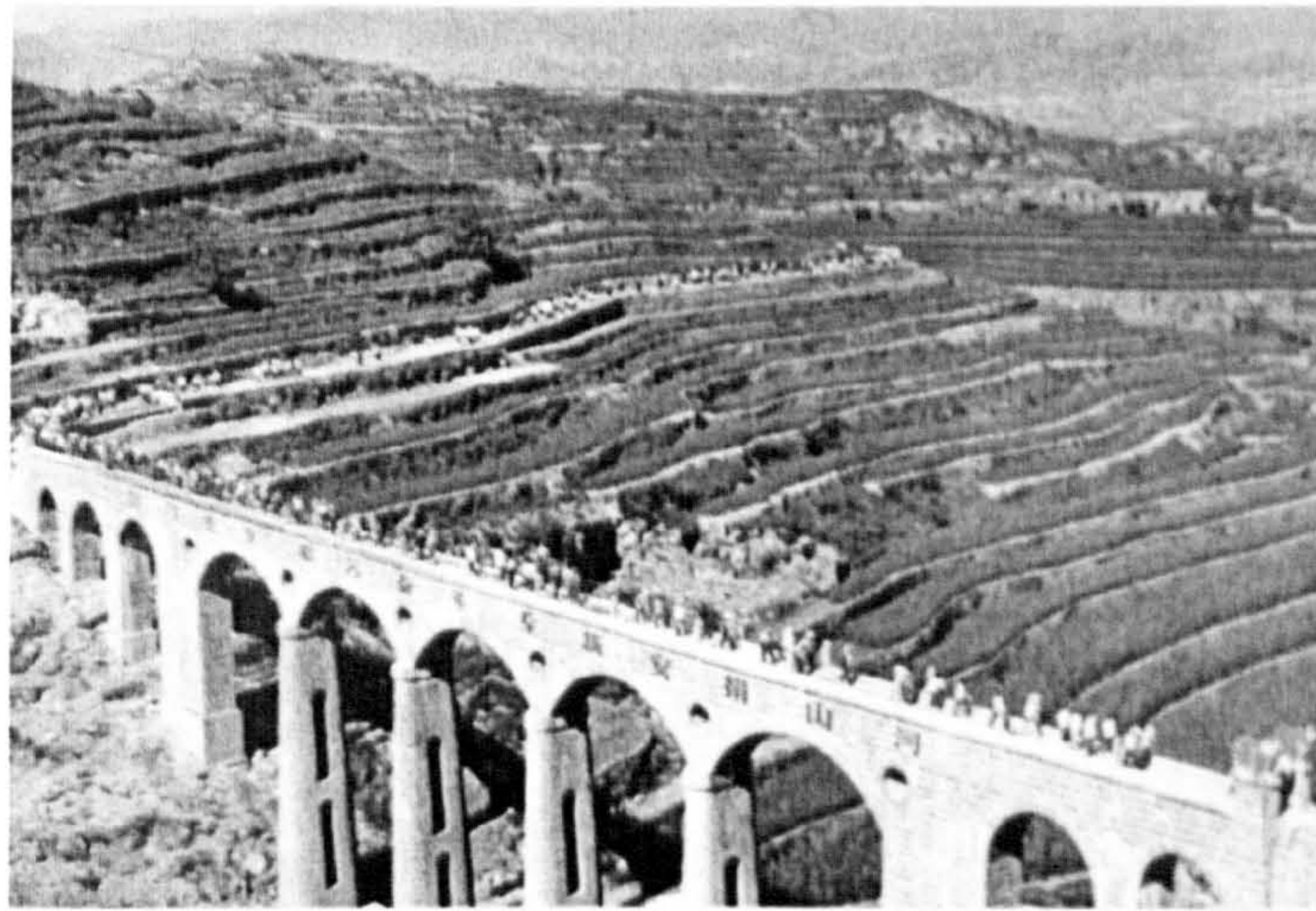
Figure 6.38 The south side of Tuanjie (Unity) Gully Aqueduct constructed in 1974, with slogan printed on facade, stating 'Ziligengsheng, jiankufendou, chongxin anpai shanhe (With self-reliance and hard work, re-arrange mountains and rivers)'.
