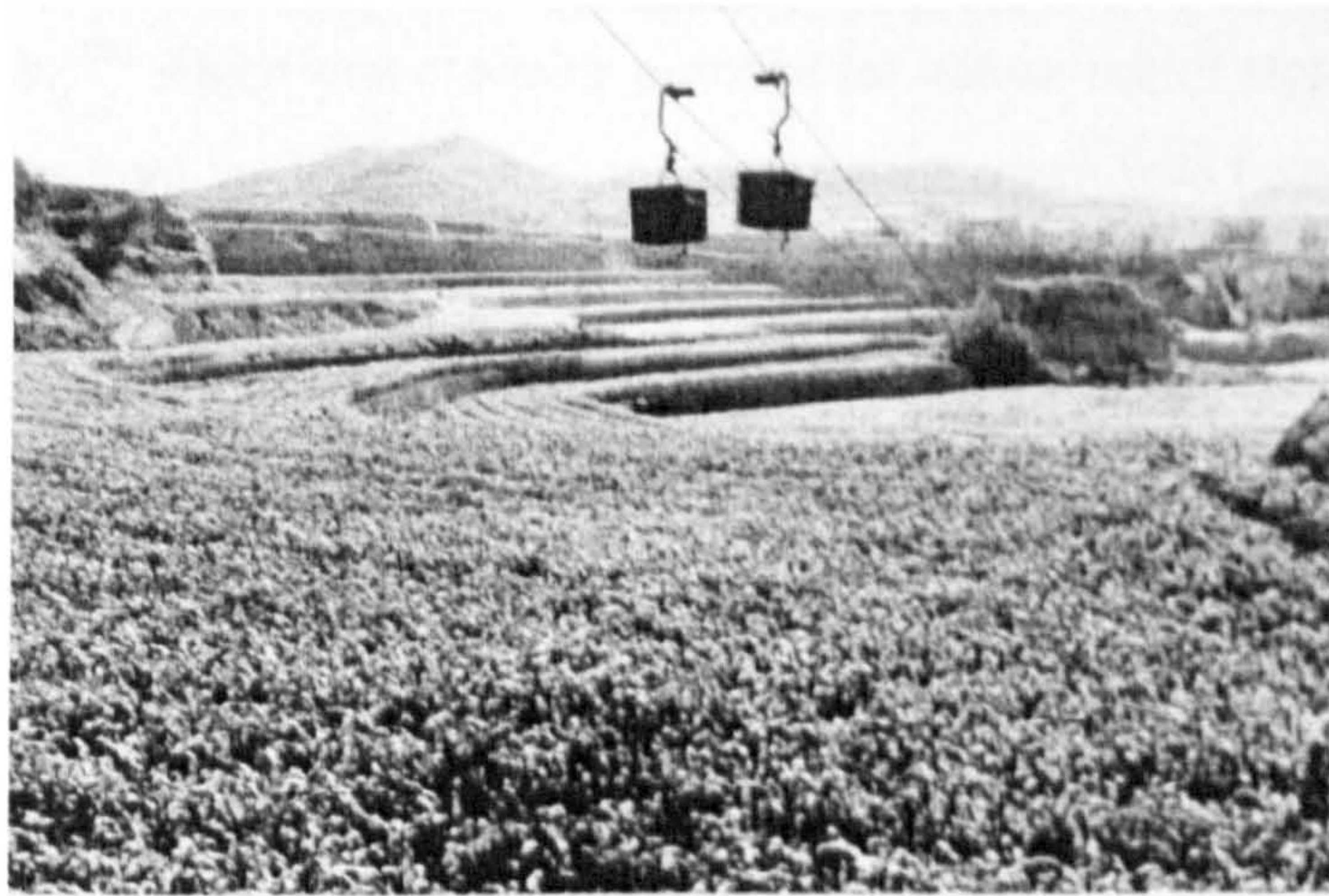
Figure 6.33 The first section of aerial cableway installed in 1967 for the purpose of transportation of stone, earth and manure. Source: supplied by Ren Zhiming.
