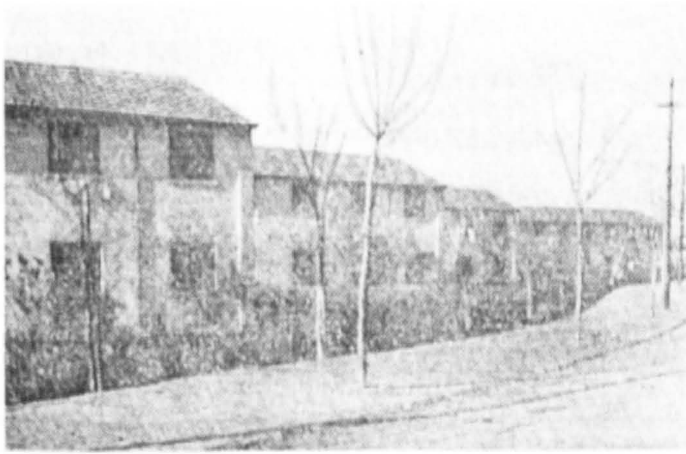
Figure 4.5 A view of Caoyang New Village, Shanghai, in mid-1950s, taken soon after trees had been planted. Source: Wang, Dingzeng 汪定曾. 'Shanghai Caoyang xinxun zhuzhaiqu de gui Hua sheji' [The planning and design of the Caoyang New Village in Shanghai] 上海曹杨新村住宅区的规划设计. Jianzhu Xuebao . 2 (1956), p. 13.
