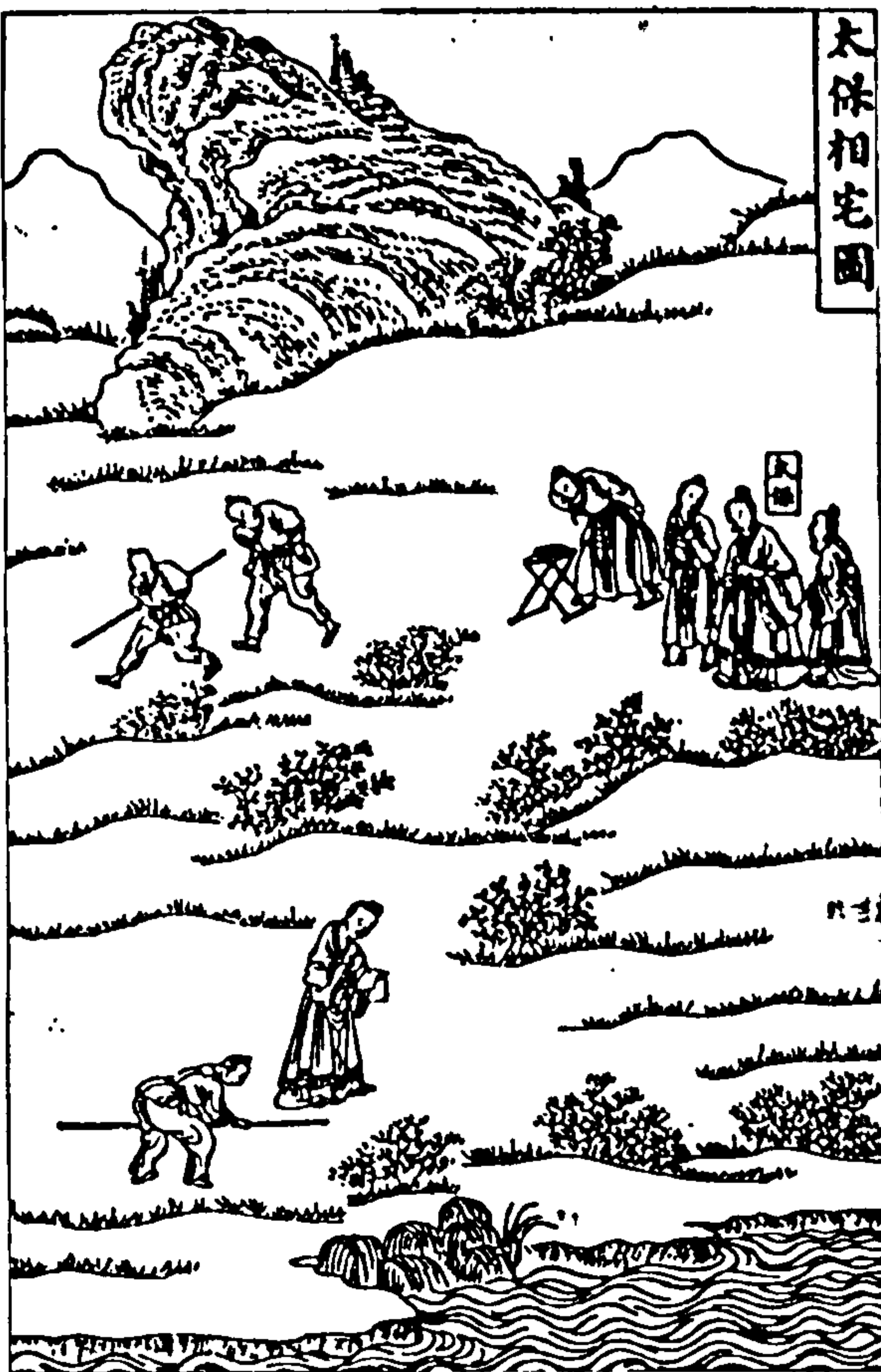
Plate 1- 10: The Situation of Tai Bao' s Site Selection and Survey in the Zhou Period, 太保相宅圖, Drawn After Literal Scripture and Visual Illustrations, 1900, Compiled and Edited by Qing Government.
