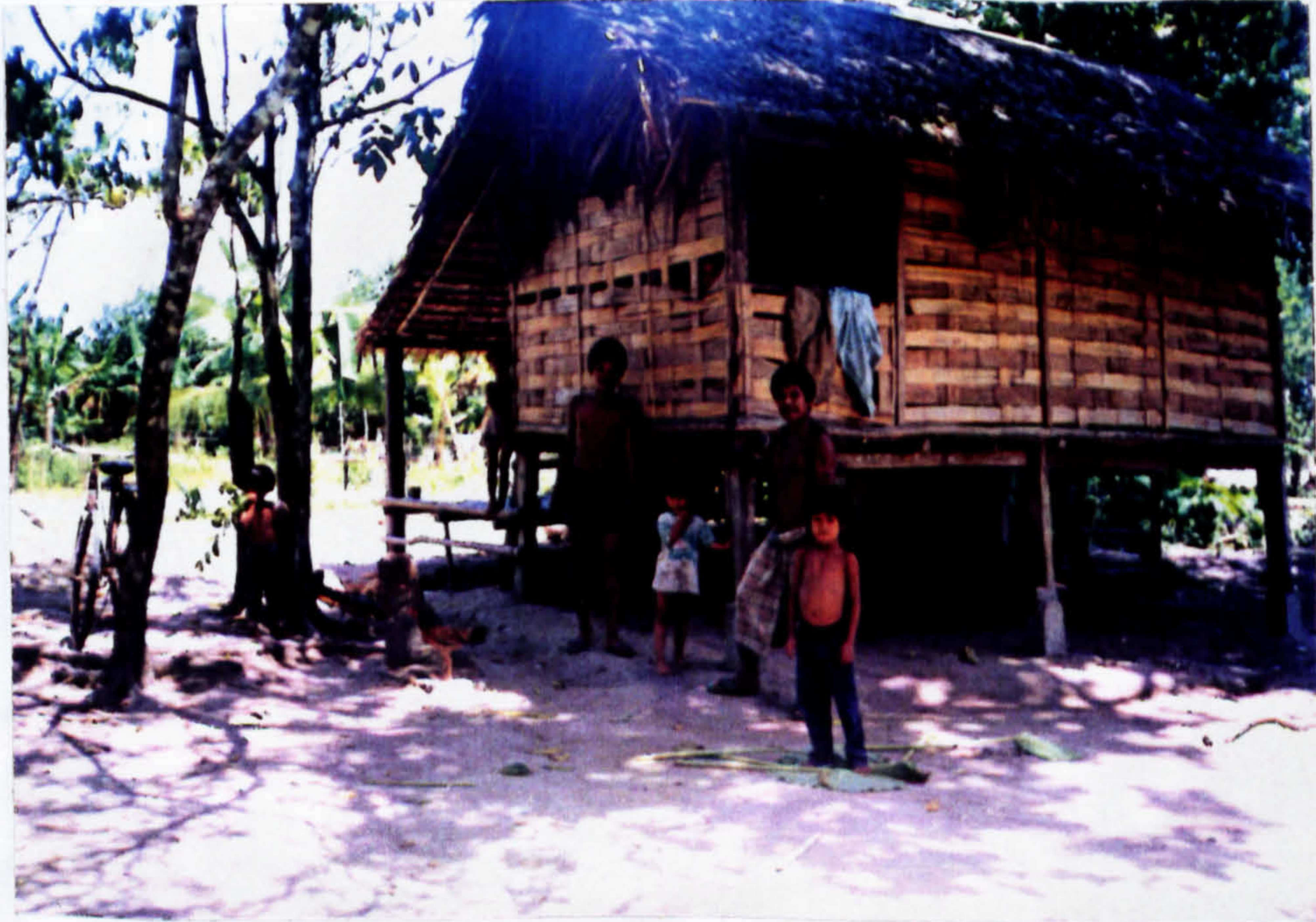
Plate K : House of peasant : Attap and bamboo wall. This type of house is generally seen as "below average" in terms of its structural conditions.
