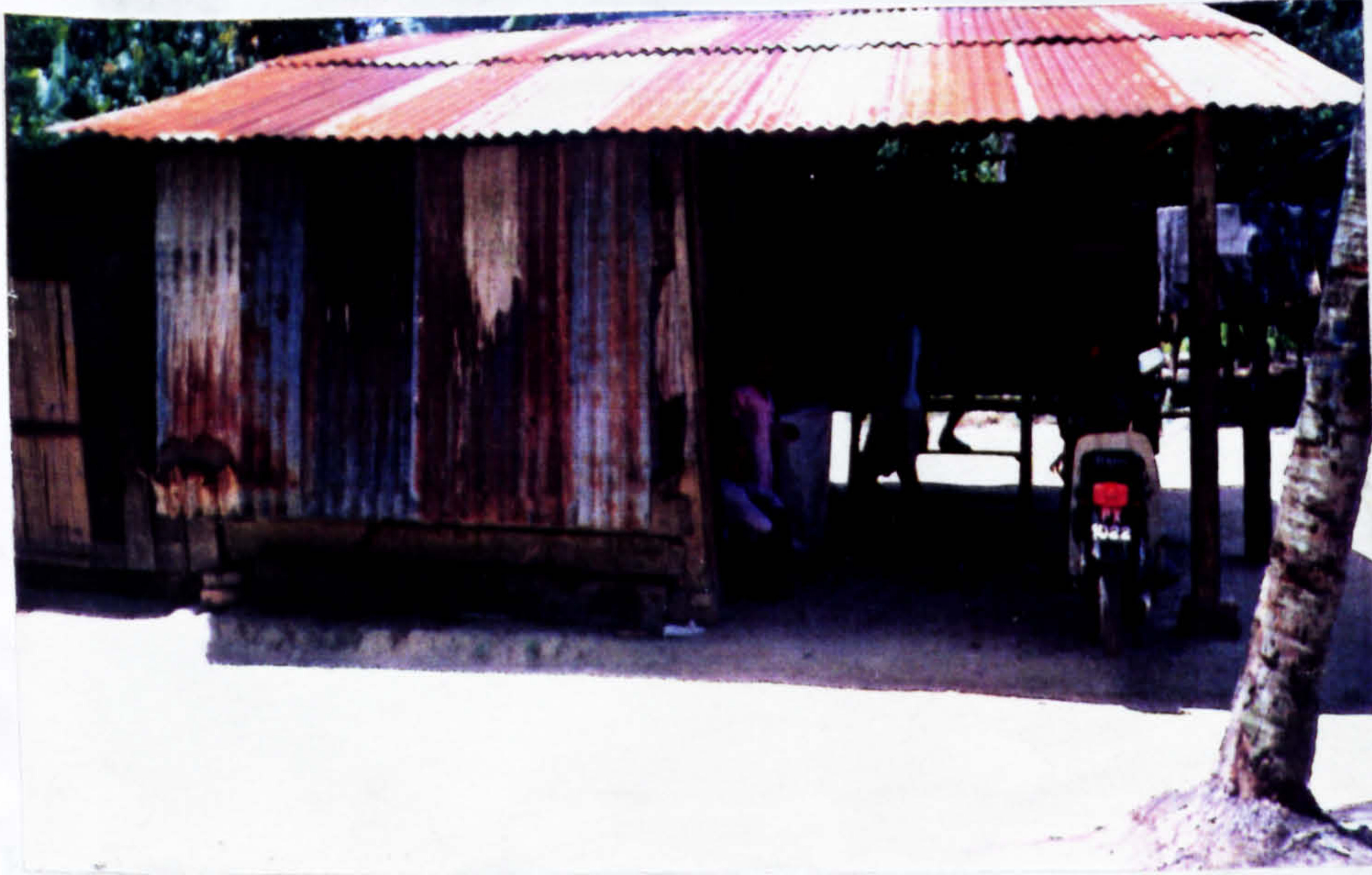
Plate J : House of peasant : Zinc wall and roof. This type of house is generally seen as "below" average in terms of its structural conditions.
