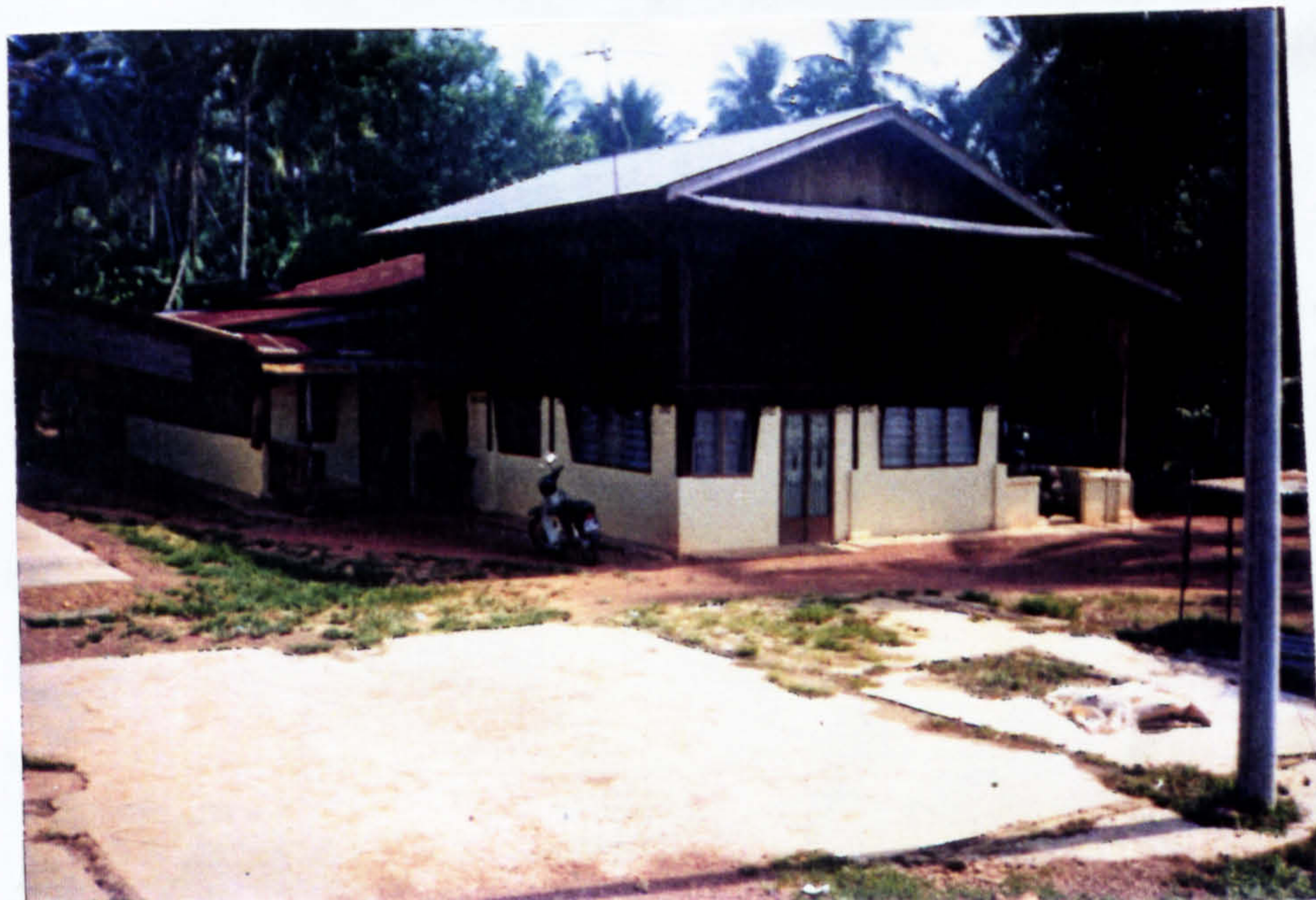
Plate P : A house normally associated with the "better off" or rural elite. Generally seen as firm in terms of its structural condition.
