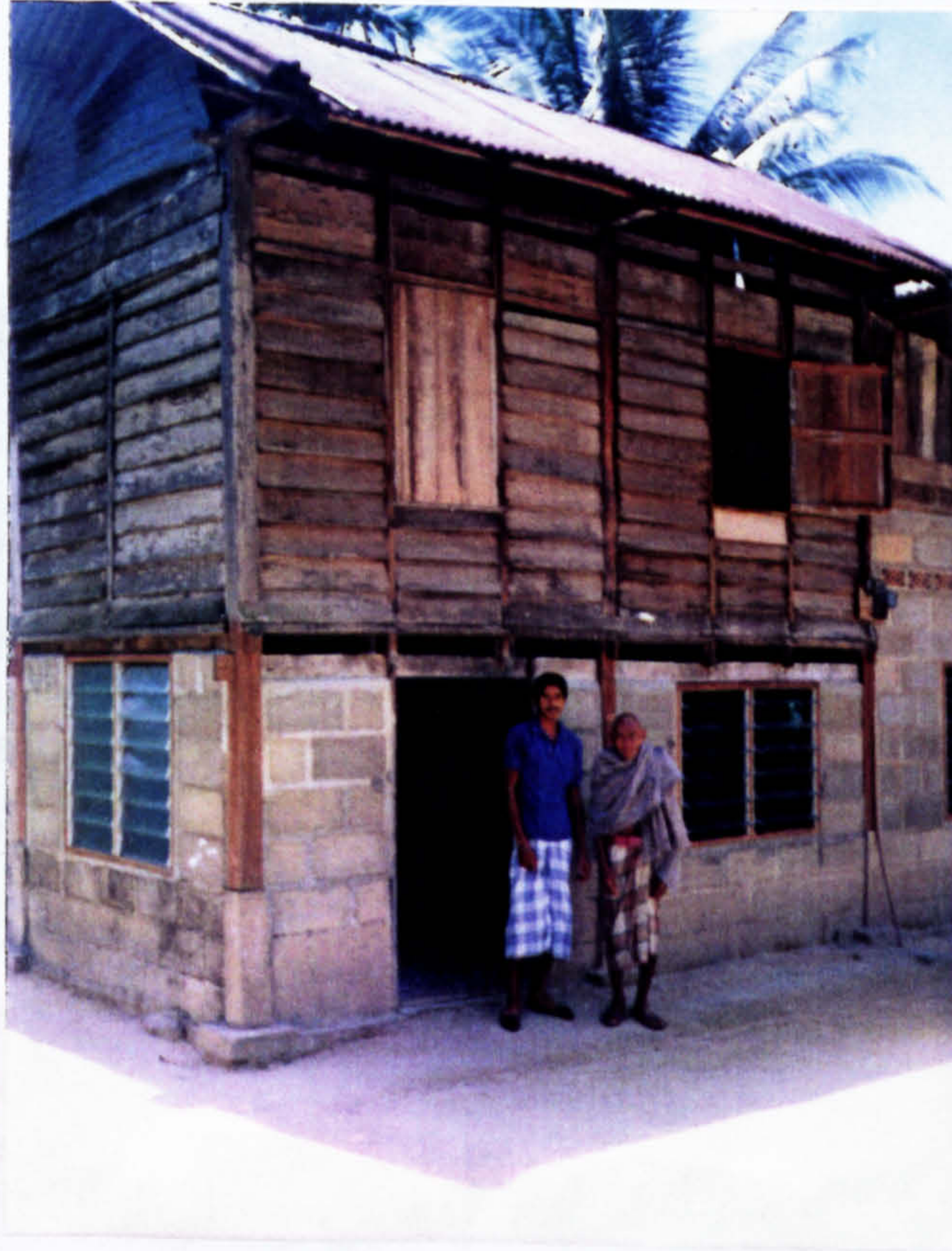
Plate N : House of peasant (double storey) : Mixtures of wooden/cement block wall and zinc roof. This type of house is generally seen as "firm" in terms of its structural condition.
