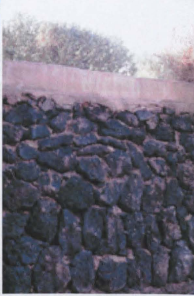
Figure: 6-1, the historic techniques of stone masonry, top, have not been studied in a way that could have inspired the modern use of stone in buildings, middle and bottom. The horizontal placement of the longitudinal side of stones, the use of takhshinah to settle stones, the carving of the outer facet of stones are all historically part of stone masonry craftsmanship in Medina. In modern practice, stones are laid vertically, with no takhshienah , and un-carved.
