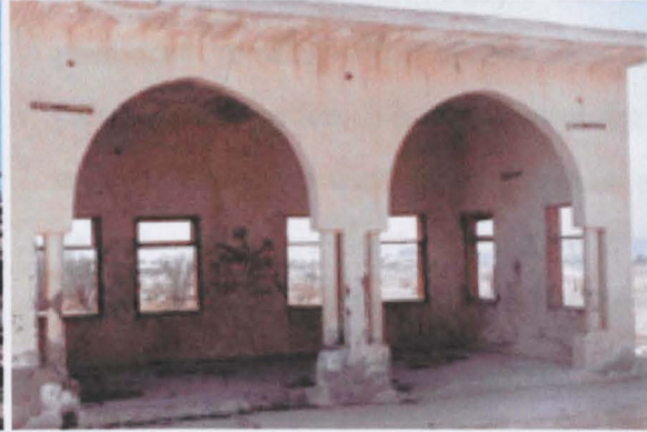
Figure: 4-23, ruins of 1970s diwans (of bilad Ali Shokri) followed almost the same morphology of Medina historic diwans. The diwan open toward the birkah through two pointed arches.
