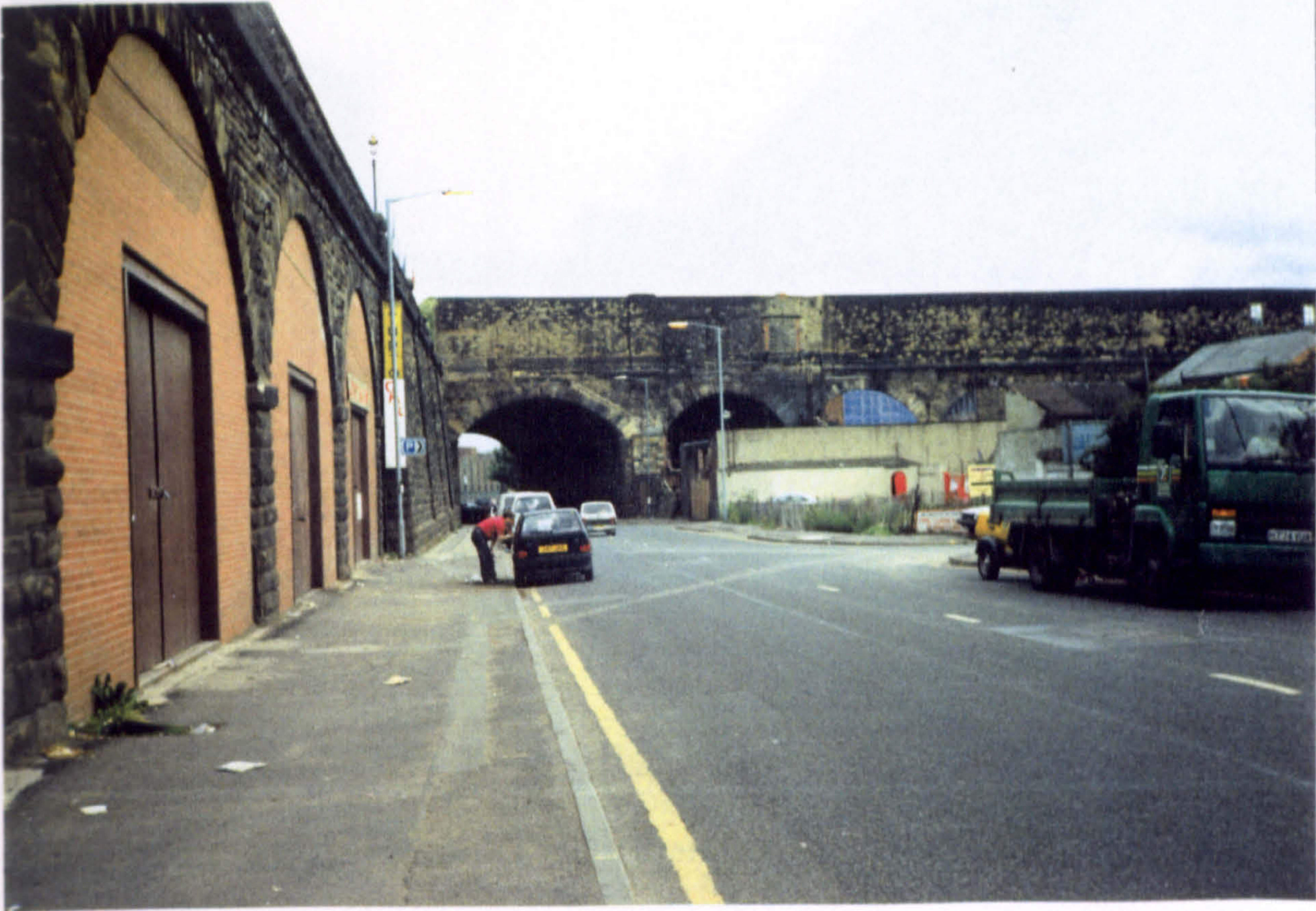
Photo 5.3: Railway Bridge Over Furnival Road (B6073)
