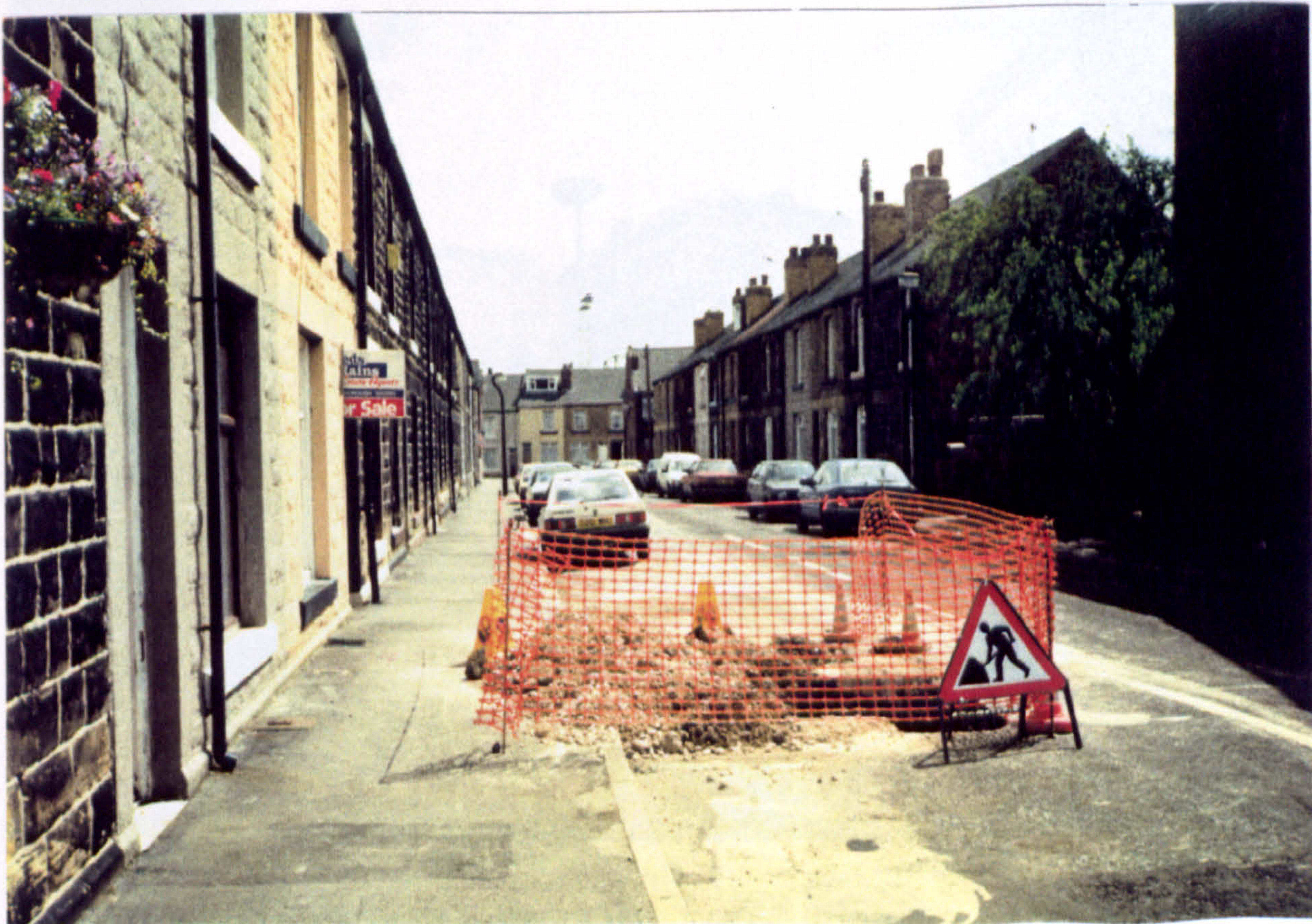
Photo 2.4: Dense Terraced Housing - Hillsborough
