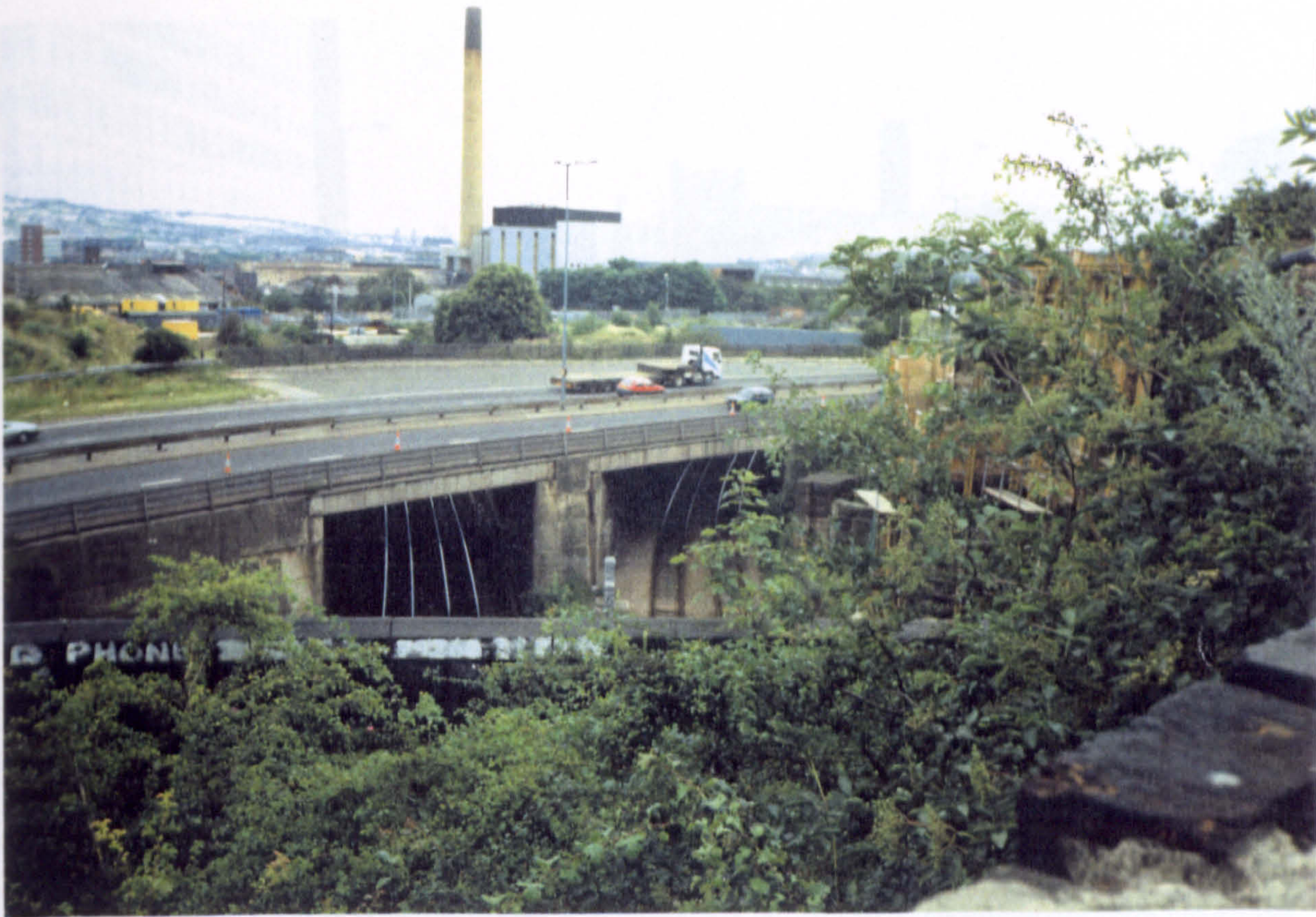
Photo 5.7: Sheffield Parkway (A57) Crossing Over Railway Line
