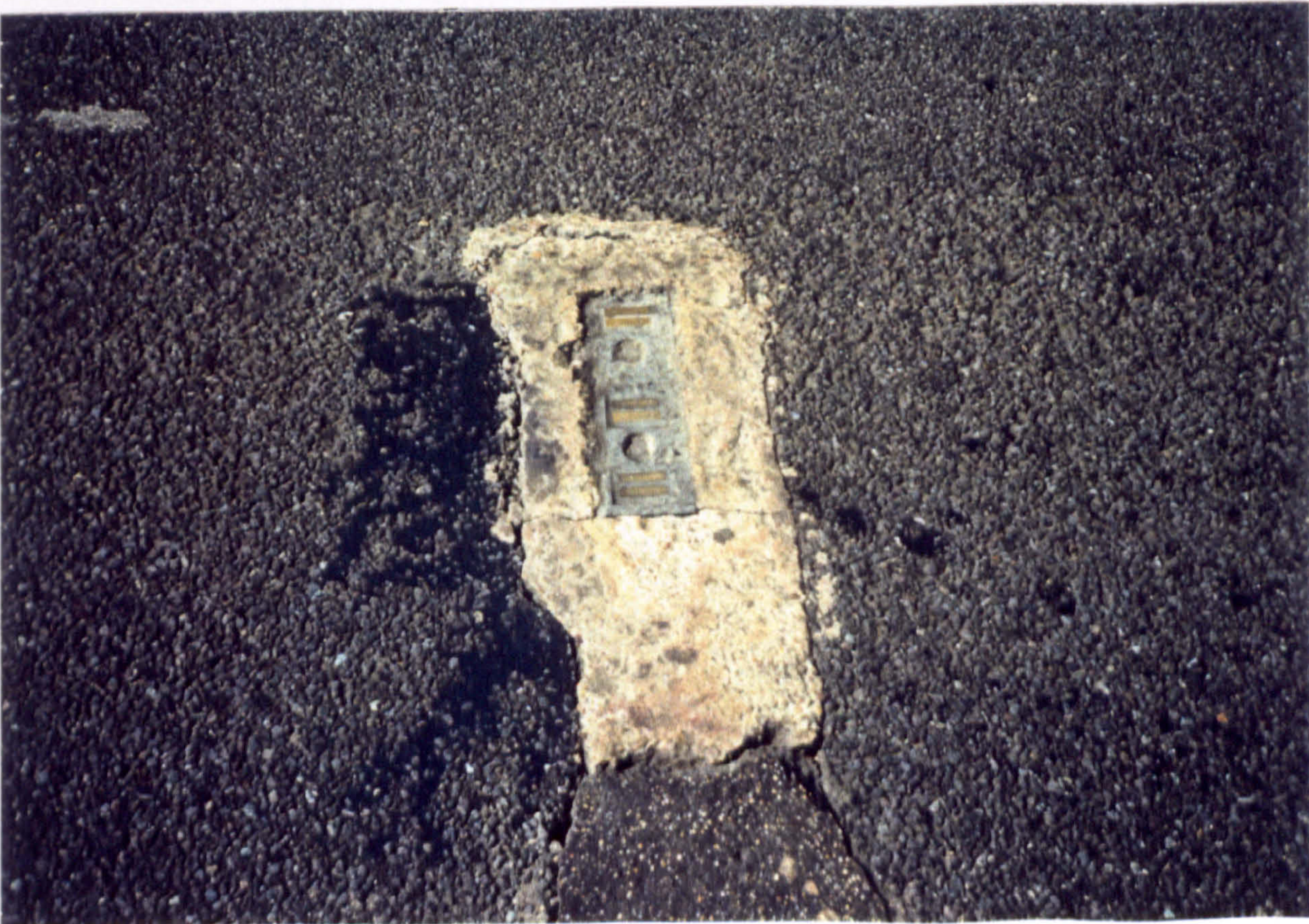
Photo 1.2: Icelert Sensor Heads Embedded In Road Surface
