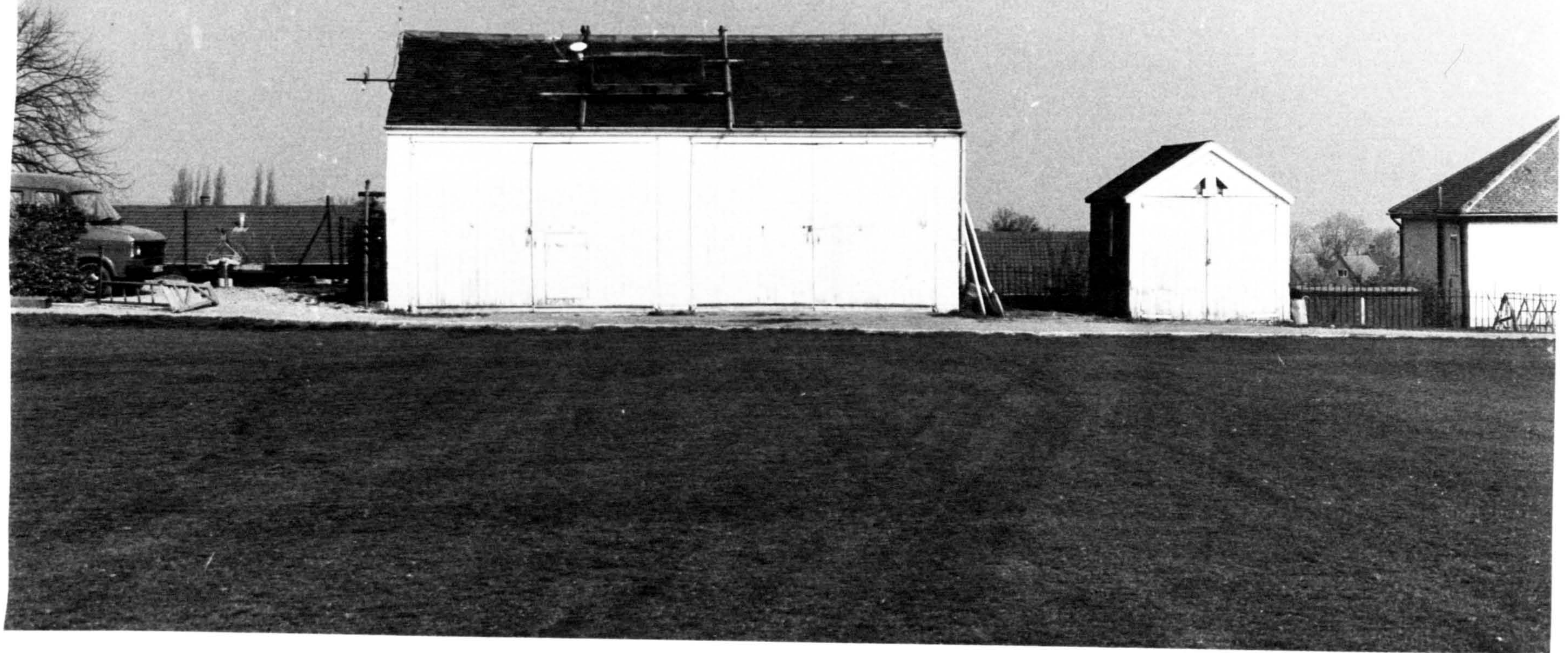
Figure 4.8 Overall view of heater plate and instrumentation mounted on the test building
