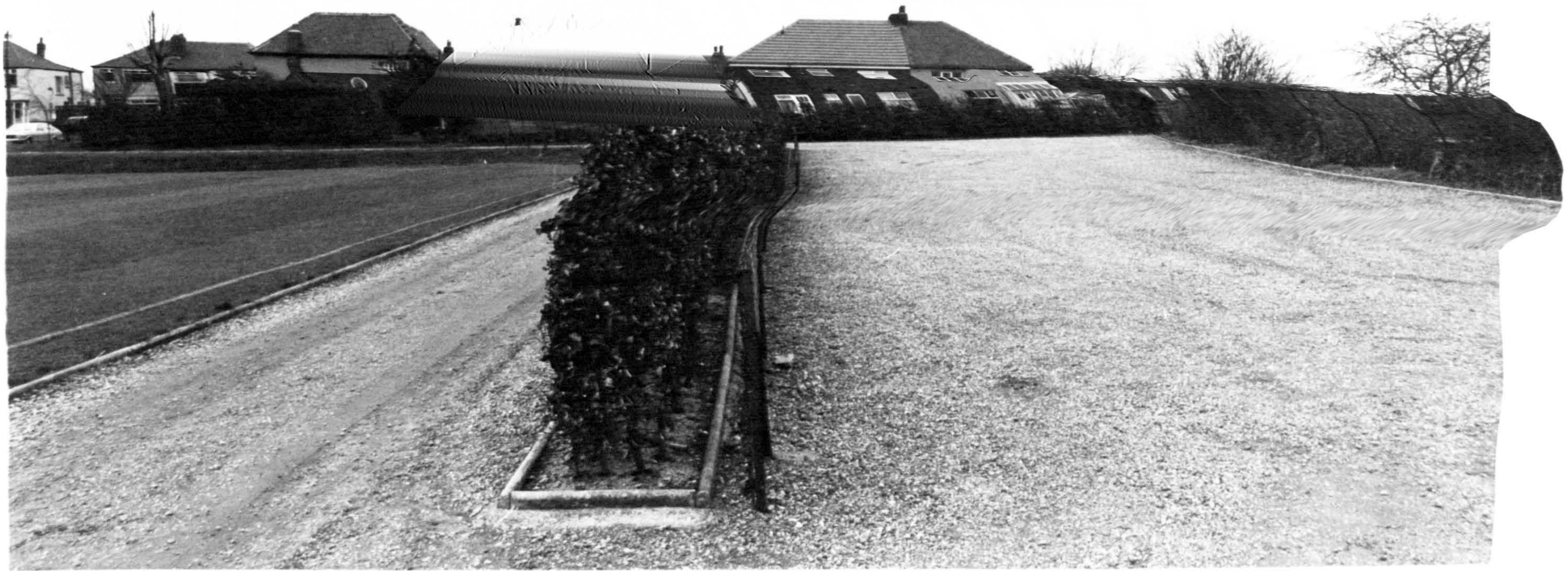
Figure 4.5 Terrain surrounding test site building - Western aspect
