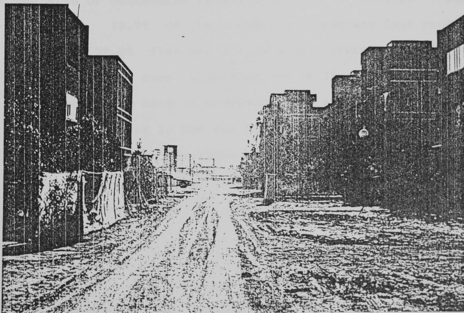
THE UNFINISHED SITE WORKS
