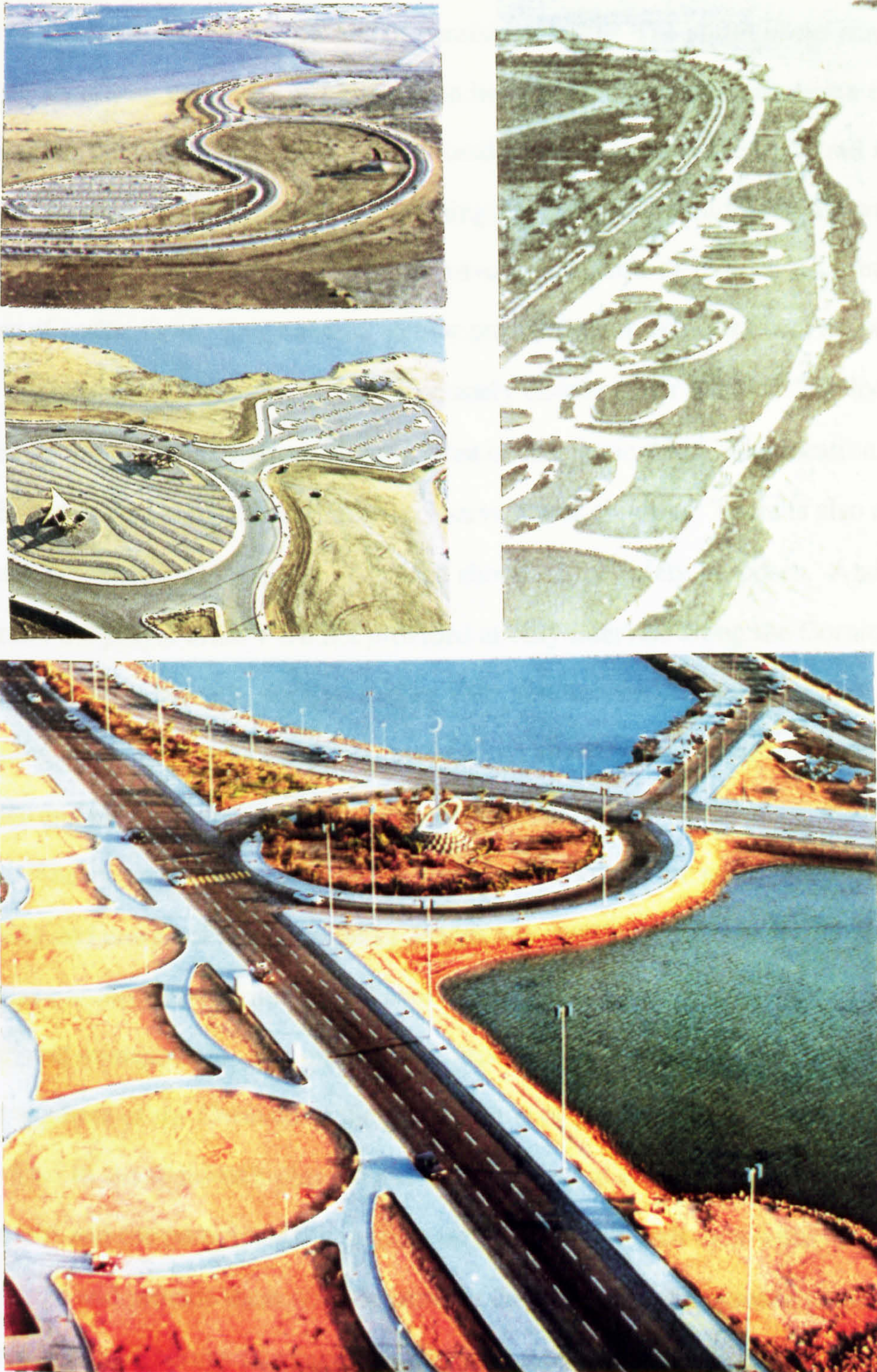
FIGURE 7.17 Many of the layouts of Jeddah's Corniche areas were shaped by meaningless geometrical patterns that were not related to the unity of design, function and purpose. Those patterns were created in these valuable urban open spaces mainly to fill the gaps and vacant lands with anything. Many of those shapes can only be appreciated in a 'birds-eye view'. 43
