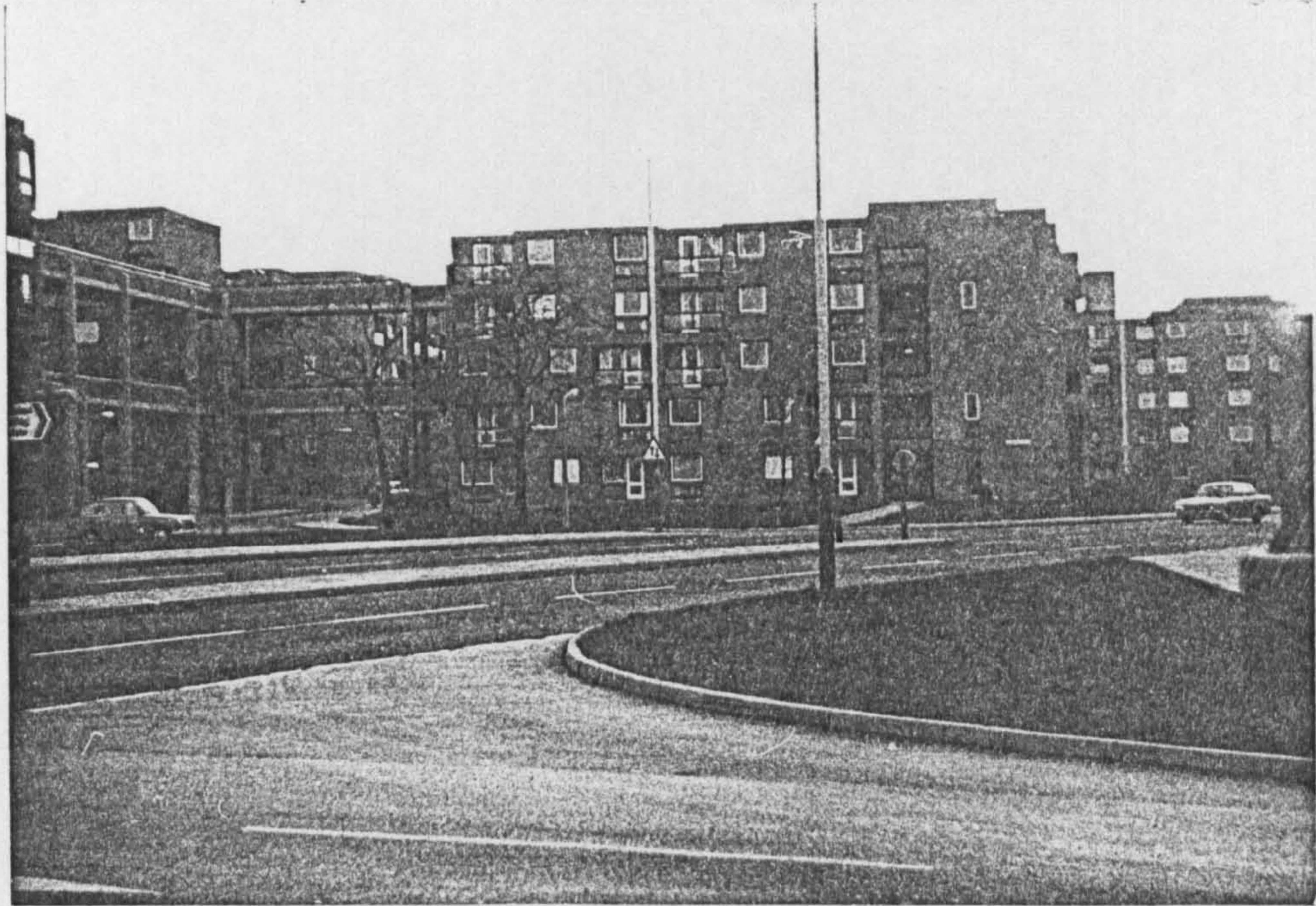
Figure 3.53 View from the main street facing the valley below.
