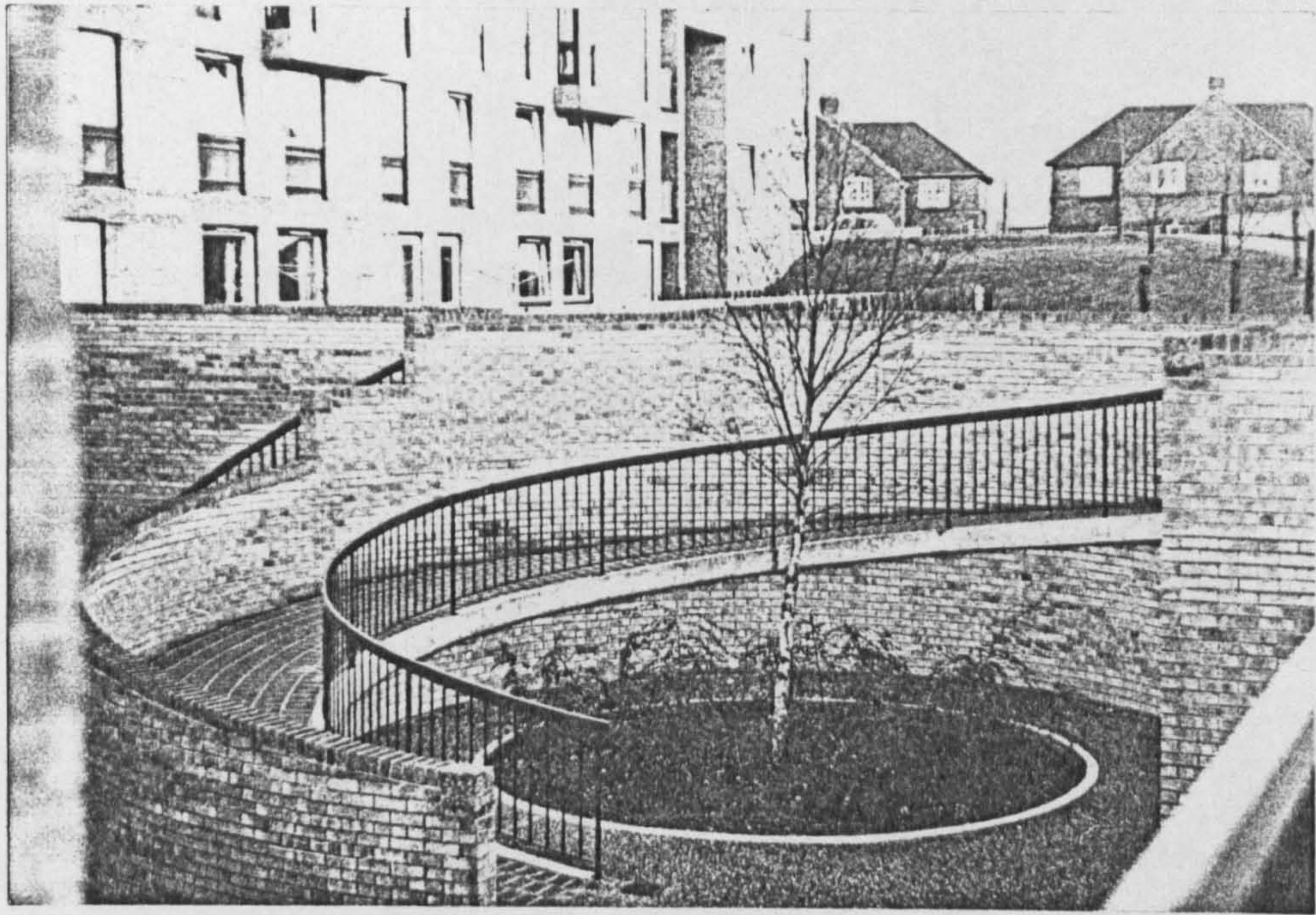
Figure 3.57 Ramp used to link two different levels in the layout.
