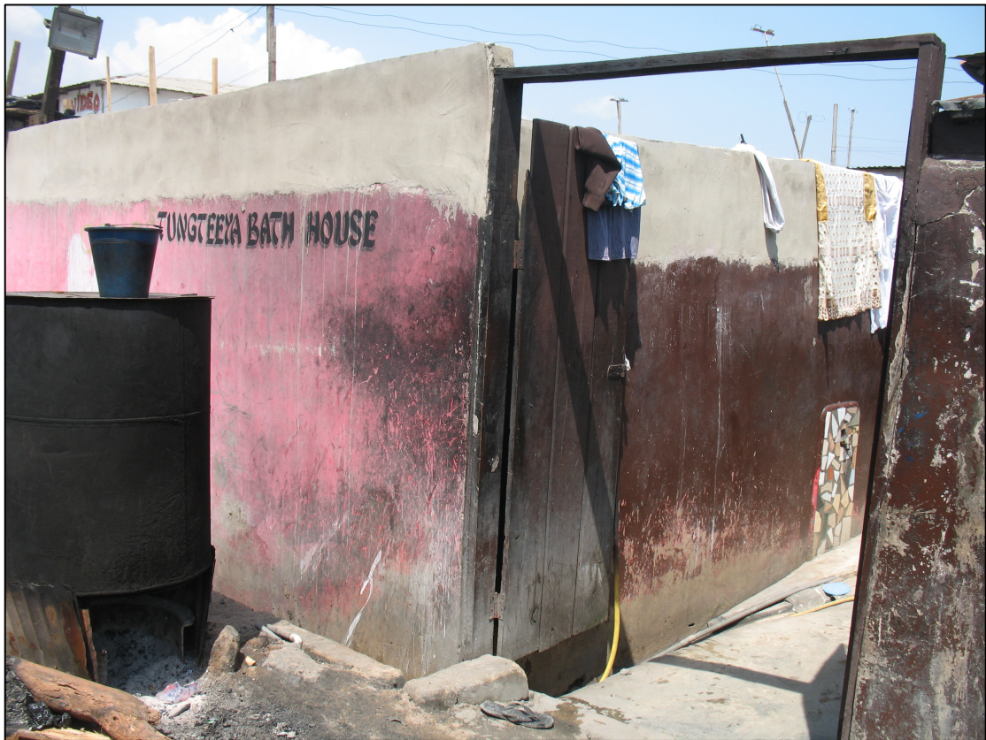
Figure 8.2: Federation-built bathhouse, Old Fadama Source: author
