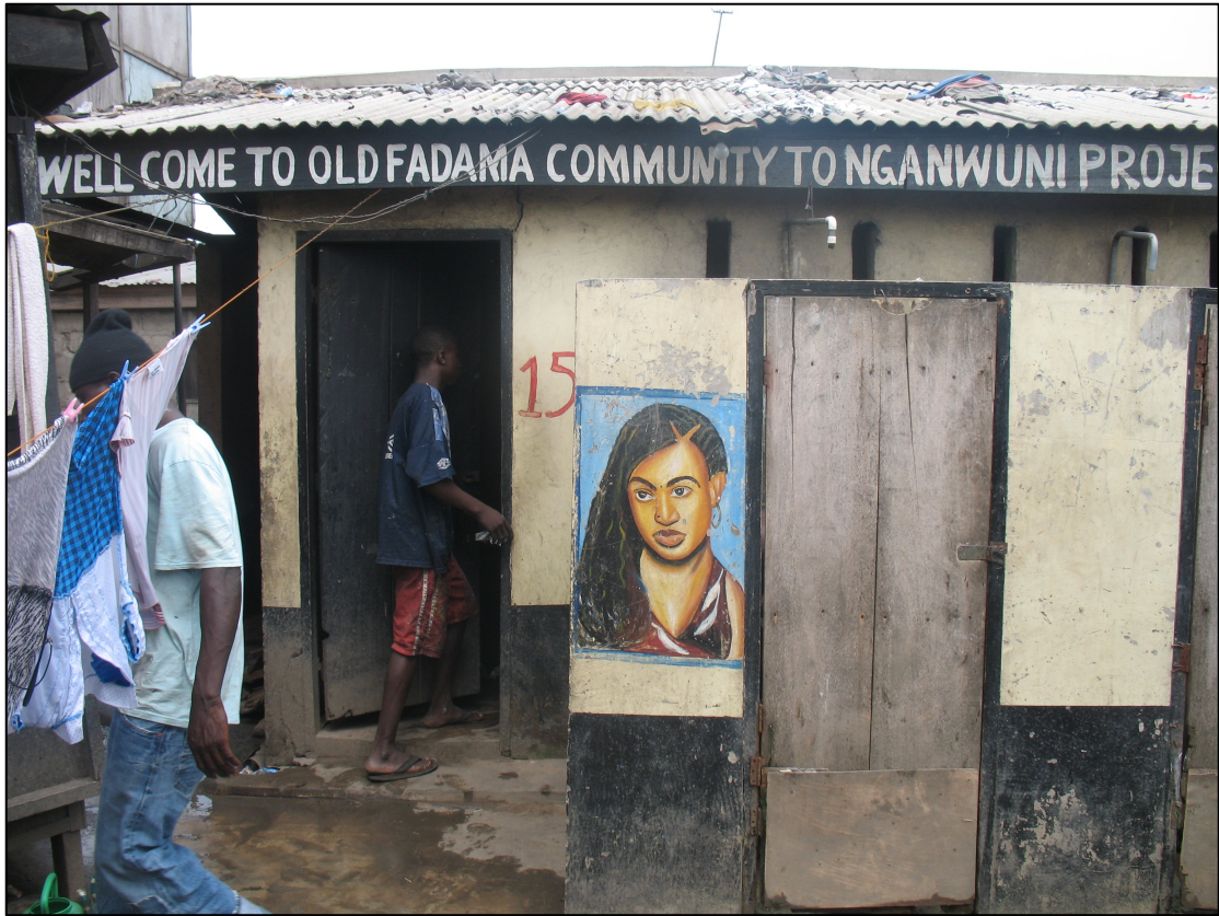
Figure 8.1: Federation-built toilet block, Old Fadama Source: author
