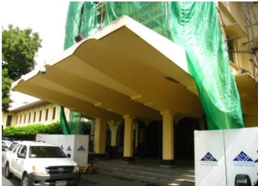
Figure 5.2.2: The reinforced concrete canopy of Thammasat University 2
