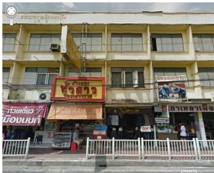
Figure 4.2.9: Typical shop houses in Thailand built during the 1940s to the beginning of 1960s applying parapets, conforming to the 1940 regulation of Bangkok Municipality 2
