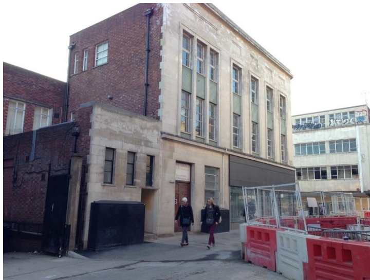
Figure 5.2.31: A corner of a building at the Moor, Sheffield, built in the 1950s shows a stone cladding façade facing the street and a normal brick façade at the rear side. 2
