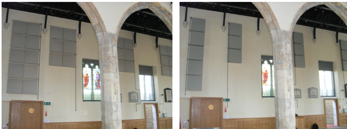
Figure 5.16 Acoustic panels set at the north wall. The 28 square absorbing panels (on the left) are folded in half, replaced by 14 reflecting panels (on the right).
