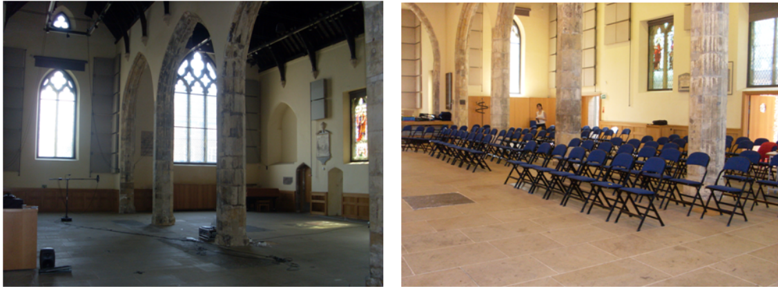
Figure 5.3 St. Margaret's Church after the refurbishment, towards the east-south (left) and the west-north (right) side of the church.
