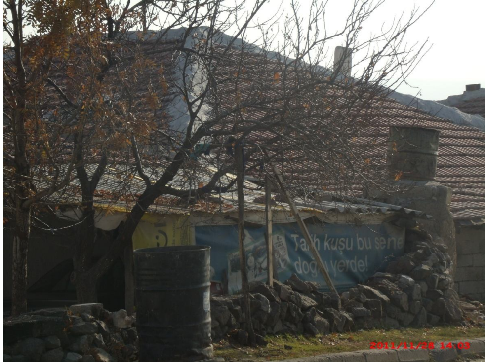
Photo 17: A gecekondu house with a chimney made from a barrel and a storage area covered with banners
