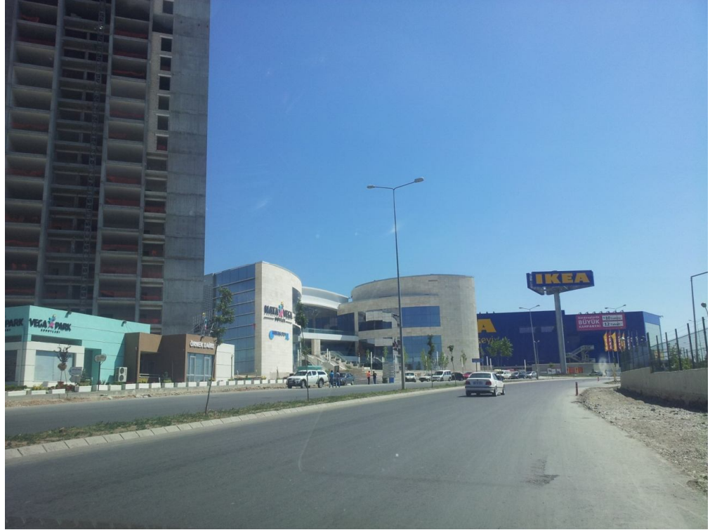
Photo 28: Looking towards the New Shopping Malls from Natoyolu Road
