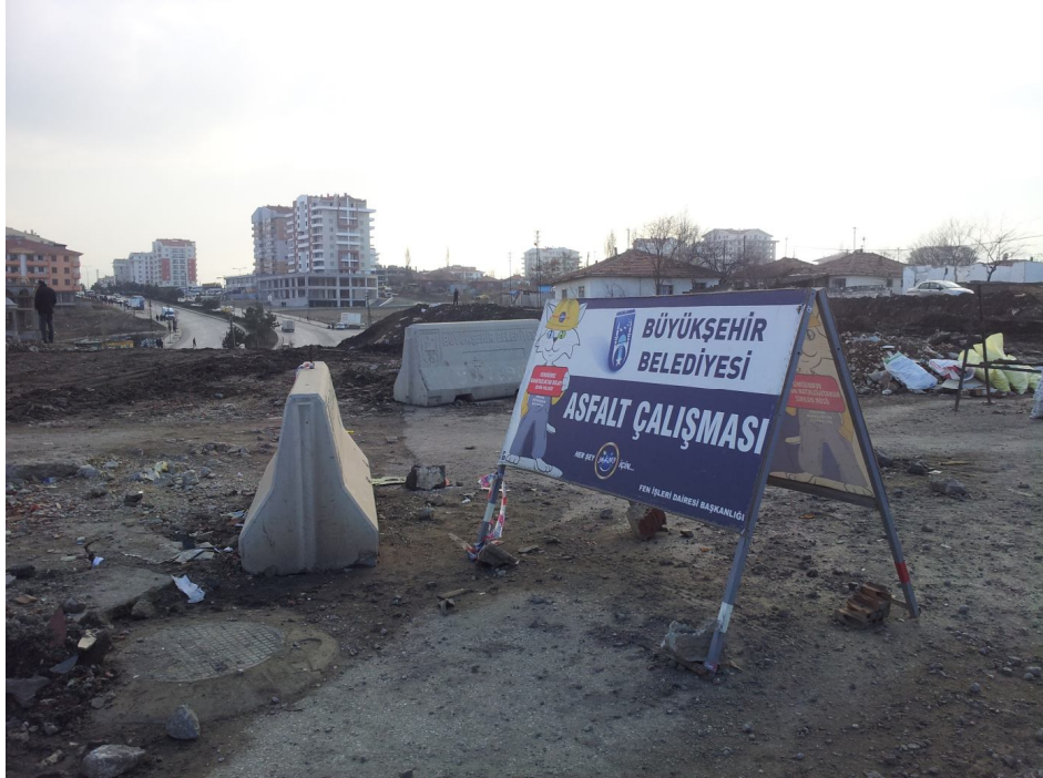
Photo 37: Ankara Municipality initiated road maintenance work after the demolition.
