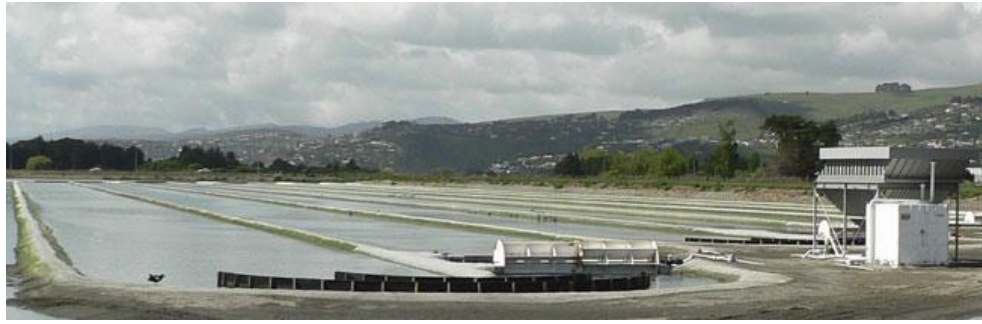
Figure 1.18 - Photograph of HRAPs in Christchurch New Zealand run by the National Institute of Water and Atmospheric Research Ltd (NIWA) (Craggs, Sutherland and Campbell, 2012)
