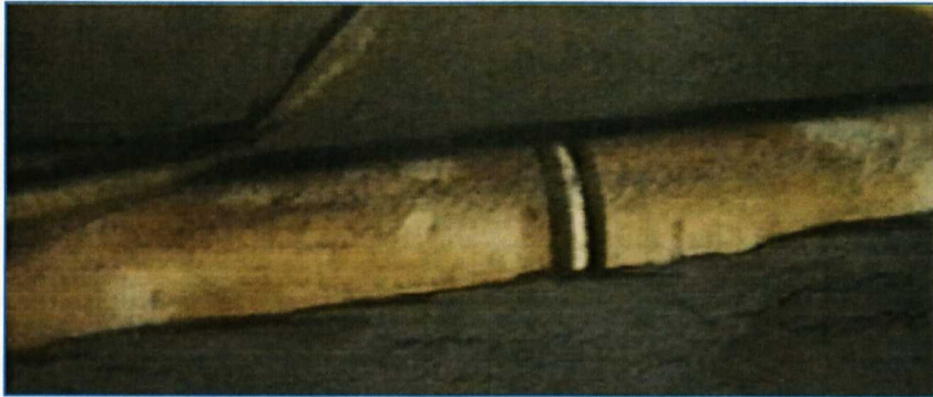
Figure 2 - 1: Typical partially embedded pipeline on the seabed
