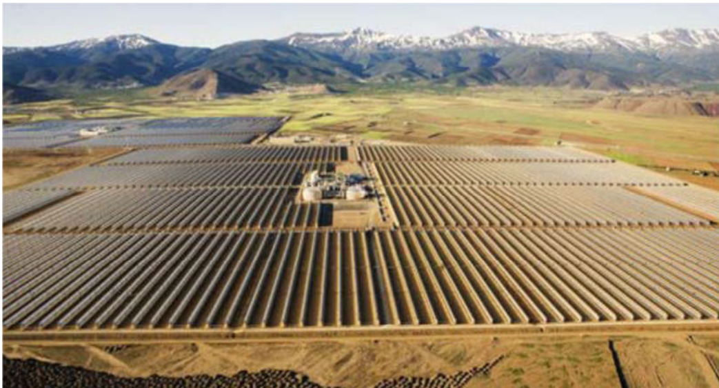
Figure 5-1: South facing view of the 50 MWe Andasol-1 Solar PTC plant in Granada, Spain (Source: [206] )
