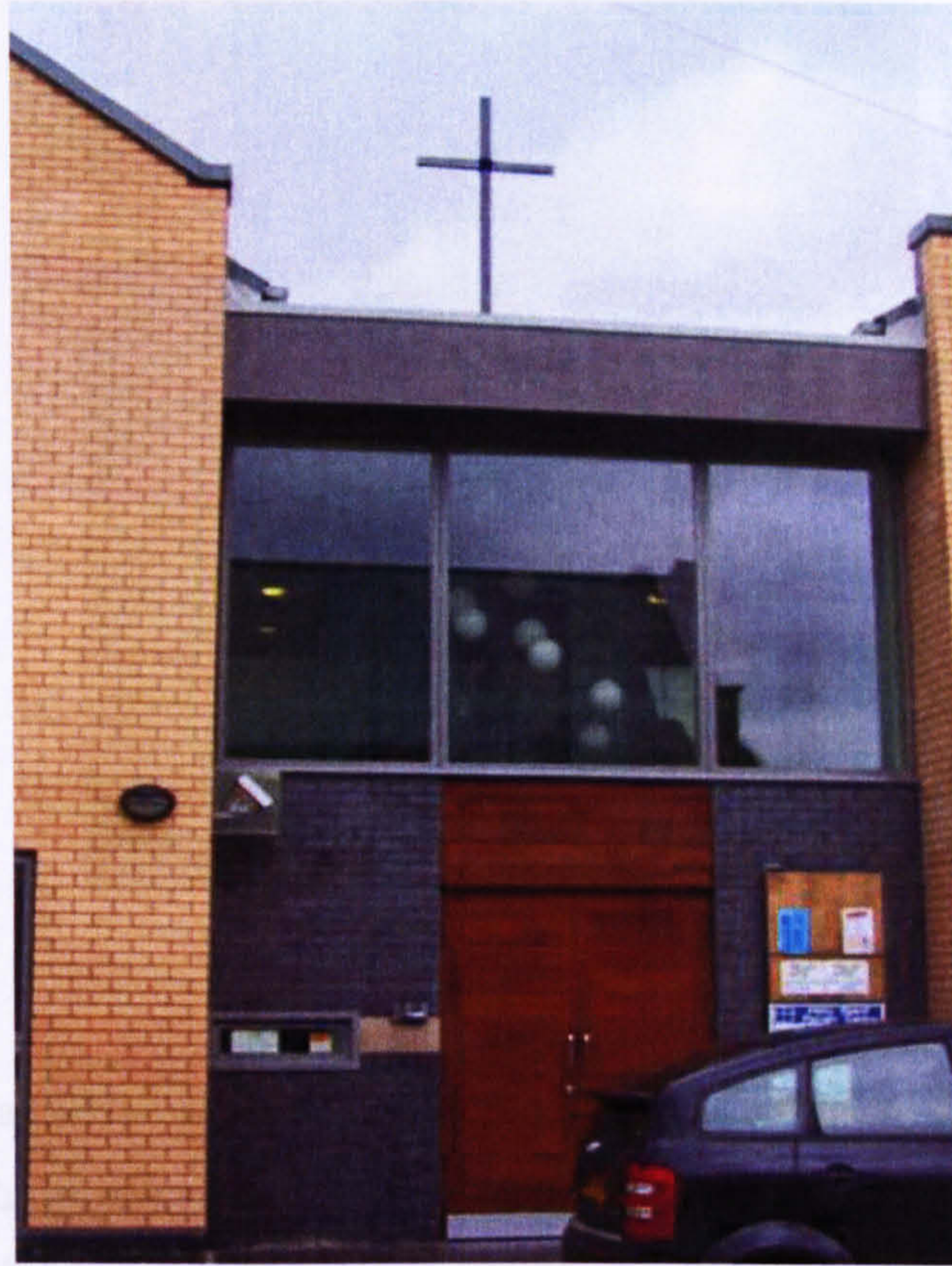
Figure 6: Photographs of the Building Blocks Crosses
