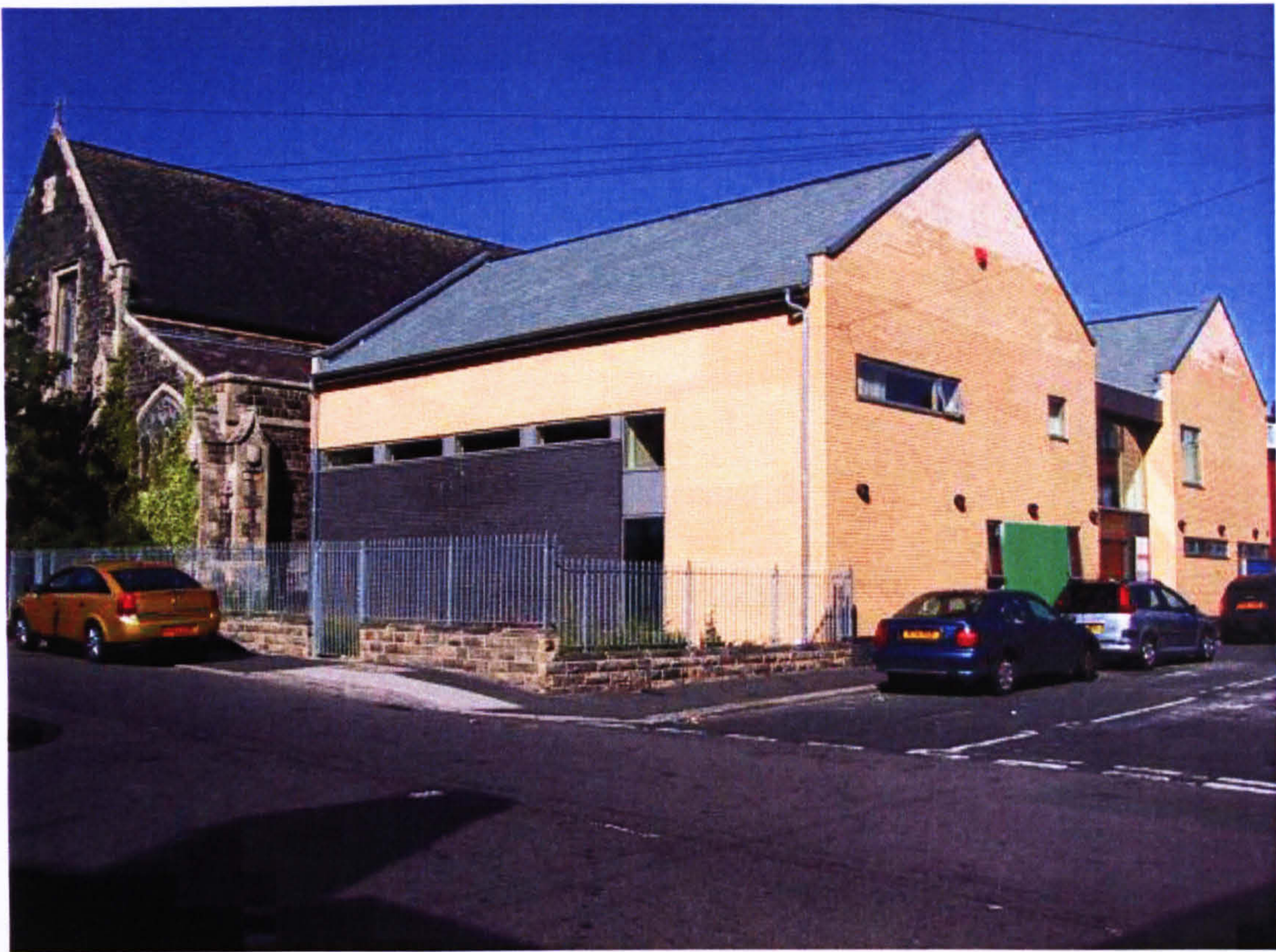
Figure 3: Photograph of the Building Blocks Centre
