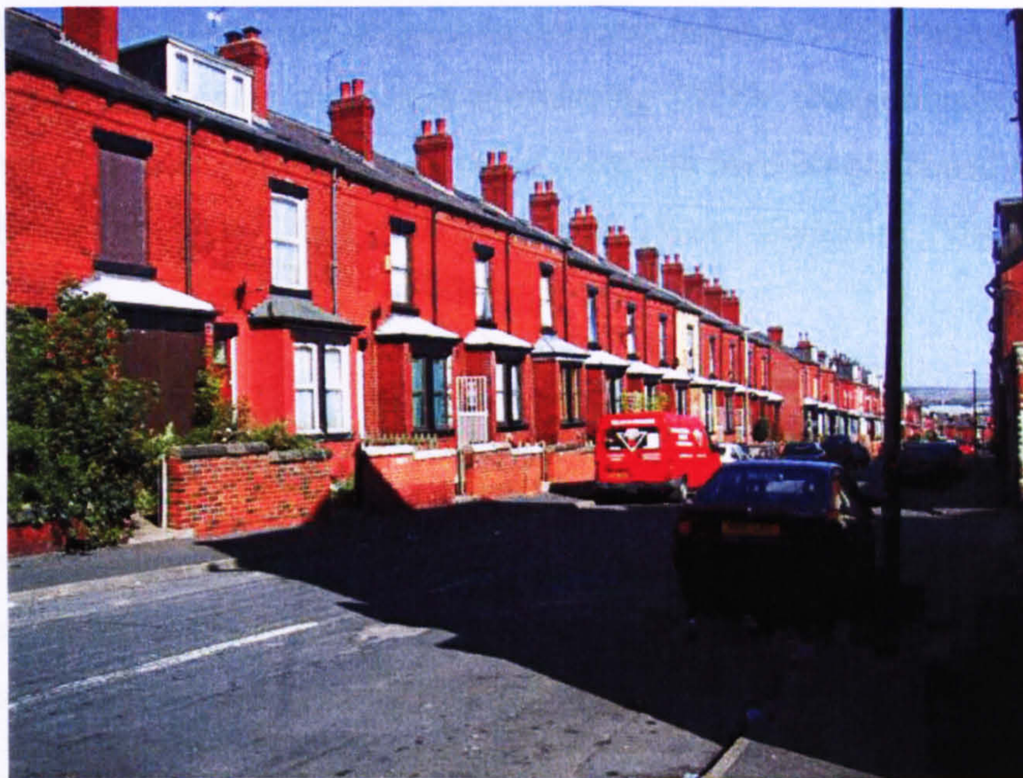
Figure 2: Photograph of a Typical Street in Beeston Hill
