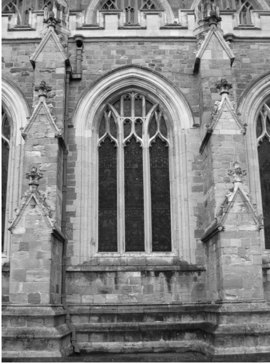
Figure 6.1: South nave aisle exterior
