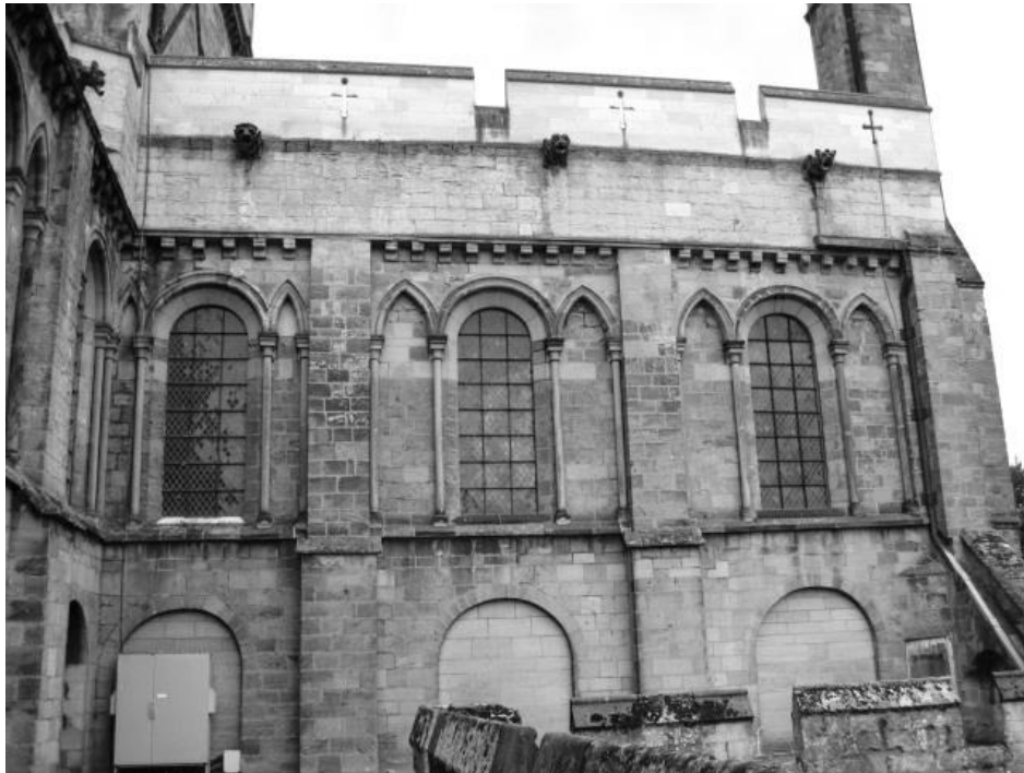
Figure 5.4: Eastern exterior of the north transept. The parapet was added after the 1450 tower collapse. Compare with Figure 5.3 to see the changes made to the east side of the south transept after 1450.
