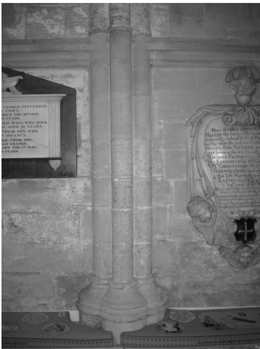
Figure 6.3: South nave aisle respond
