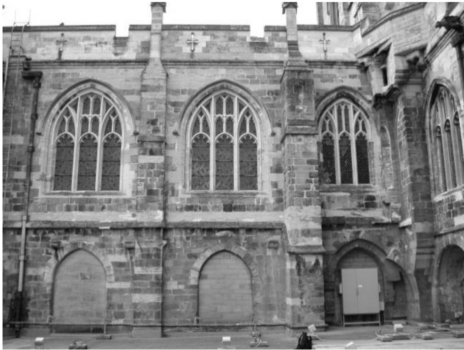
Figure 5.3: Eastern exterior of the south transept. This photograph shows the features altered or added as part of the c. 1465–1480 renovations. These include the window tracery, buttresses, and parapet. See Figure 5.4 for the c. 1175 clerestory windows, buttresses, and cornice. Note also that masonry that forms the juncture of the east wall of the transept and south wall of the choir is a damaged portion of the original c. 1175 building. The south wall of the choir clerestory was thinned well before the tower collapse, probably c. 1290.
