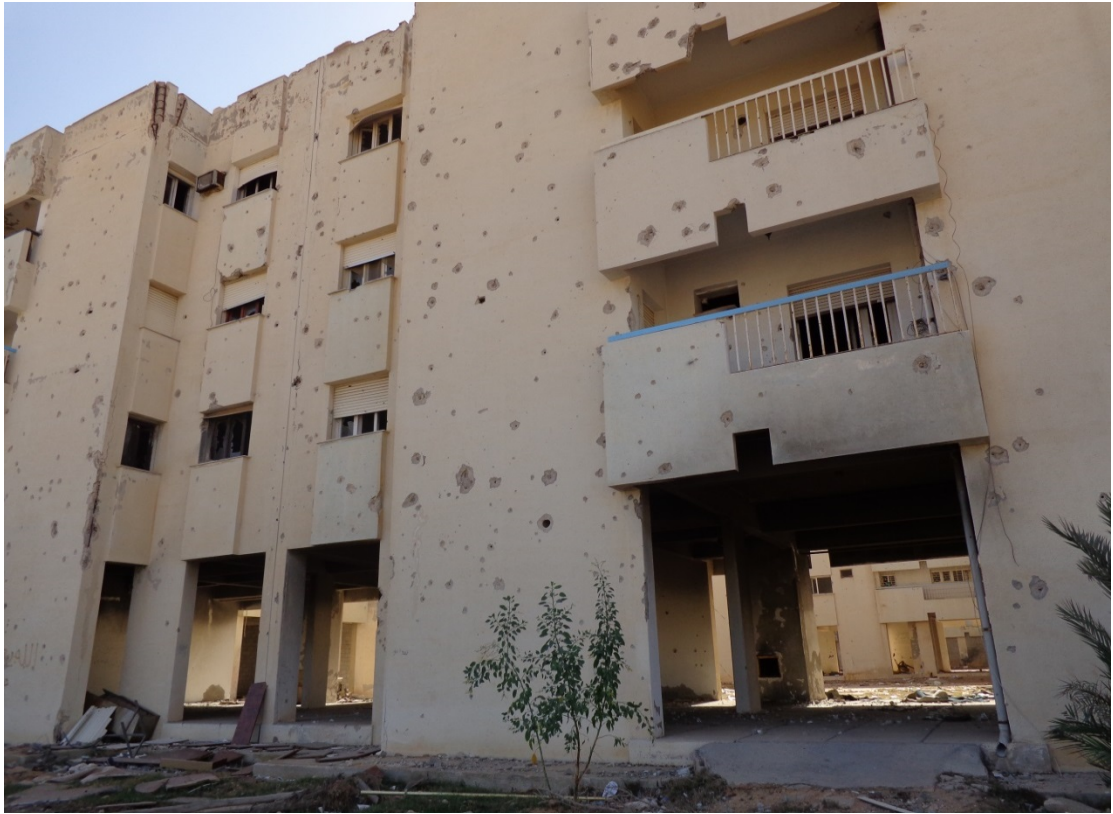
Photo F: Heavily damaged building - Faculty of Medical Technology in Misrata
