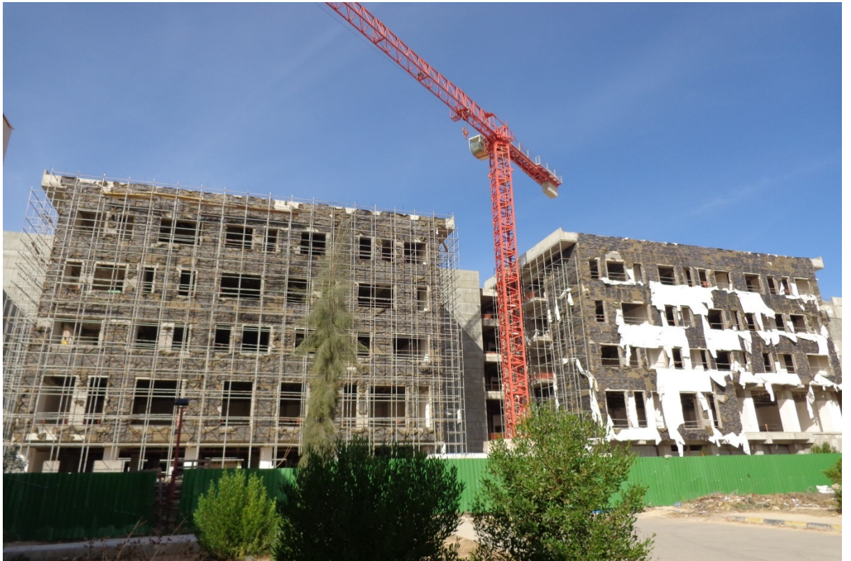
Photo A: Unfinished campus construction at Tripoli University Campus B
