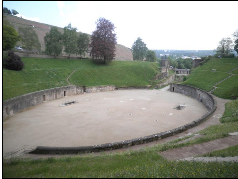
Figure 3.9: Amphitheatre in Trier as it appears today. The entrances for the cages built into the walls of the arena are visible. Copyright author.
