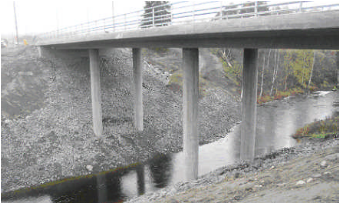
Figure 5.2: Photograph of the Haavistonjoki Bridge after construction (Kerokoski, 2006)
