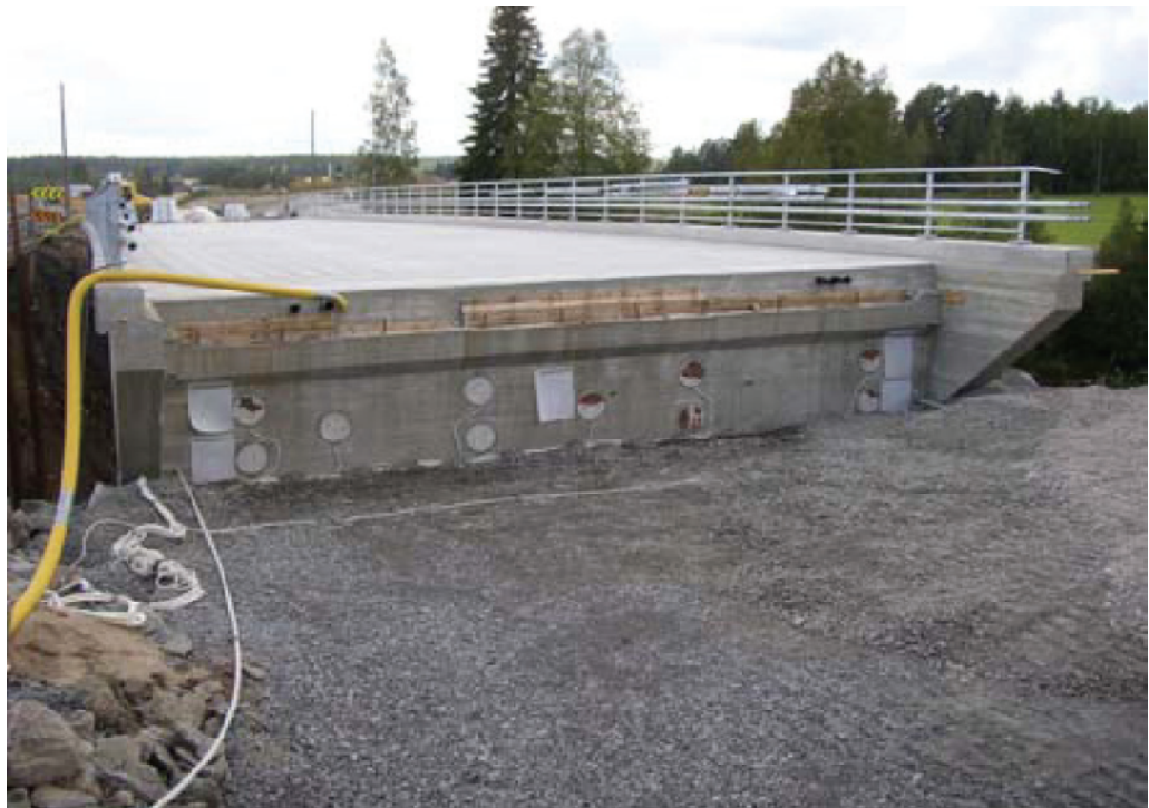
Figure 5.6: Photograph of bridge abutment showing location of earth pressure cells (Kerokoski, 2006)
