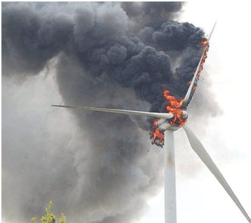
Figure 5.1: One of many wind turbines whose overheated gearbox caused fire [50].
