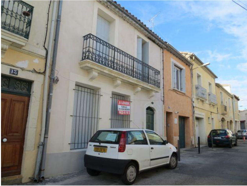
Figure 6.12: Renovated facades in the Rue du Père Fabre, in the ‘streets of saints’, November 2012. Photograph: Roza Tchoukaleyska.
