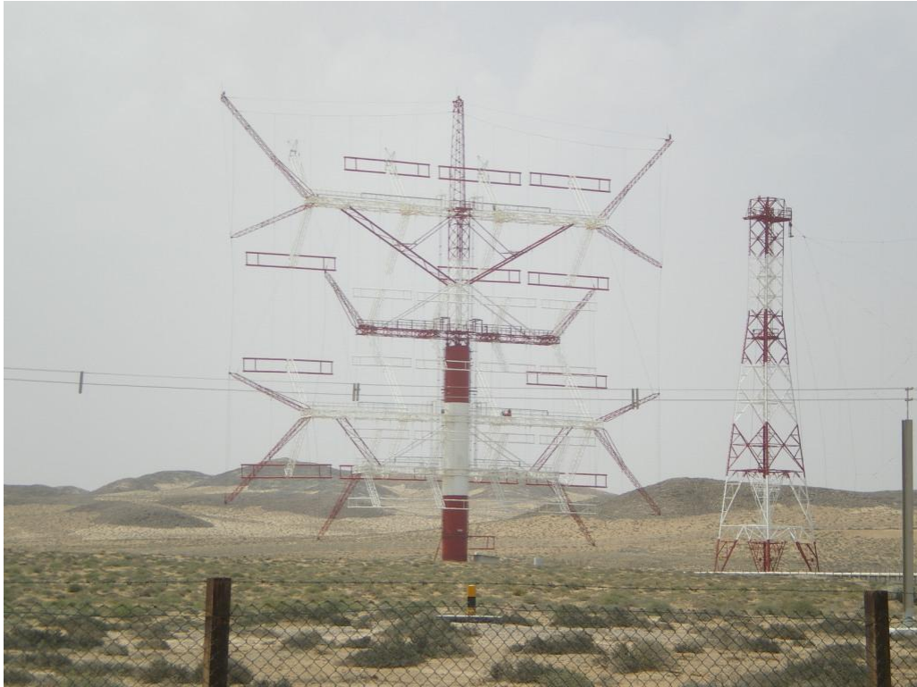
Fig 2.1 A'Seelah (Oman) Transmitting station rotatable HF curtain array
