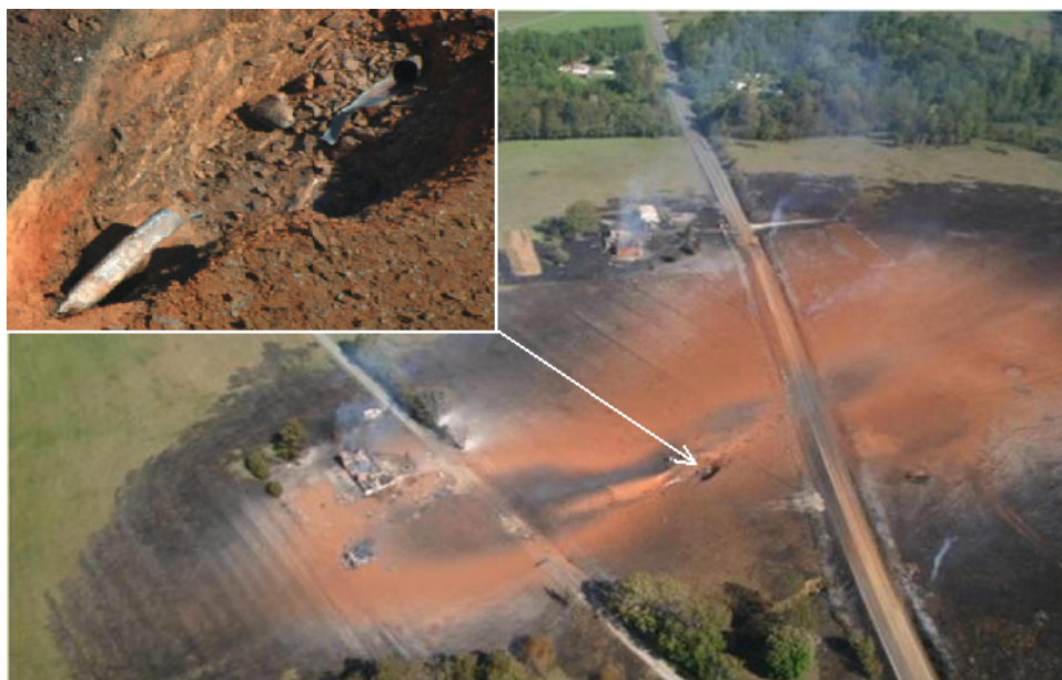
Figure 1.1: Appomattox, Virginia, USA, 2008, after a natural gas pipeline explosion [EnergyindustryPhotos, 2008]
